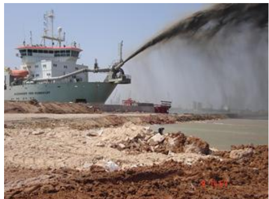
Figure 6: Repulsing of dredged material
