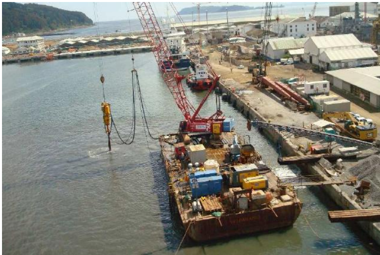
Figure 2: ASMAR Shipyard – stone column installation from the barge.
