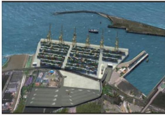
Figure 7: New Container Terminal in La Guaira Port
