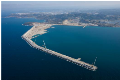
Figure 12: New outer harbour, October 2010
