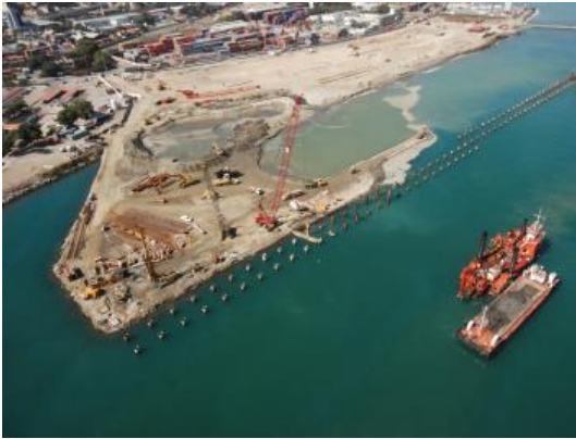
Figure 8: New Container Terminal in La Guaira Port
