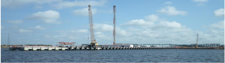
Figure 4: General overview of the works in the final stage.
