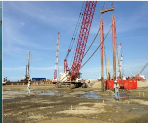
Figure 9: Execution of vibroflotation
