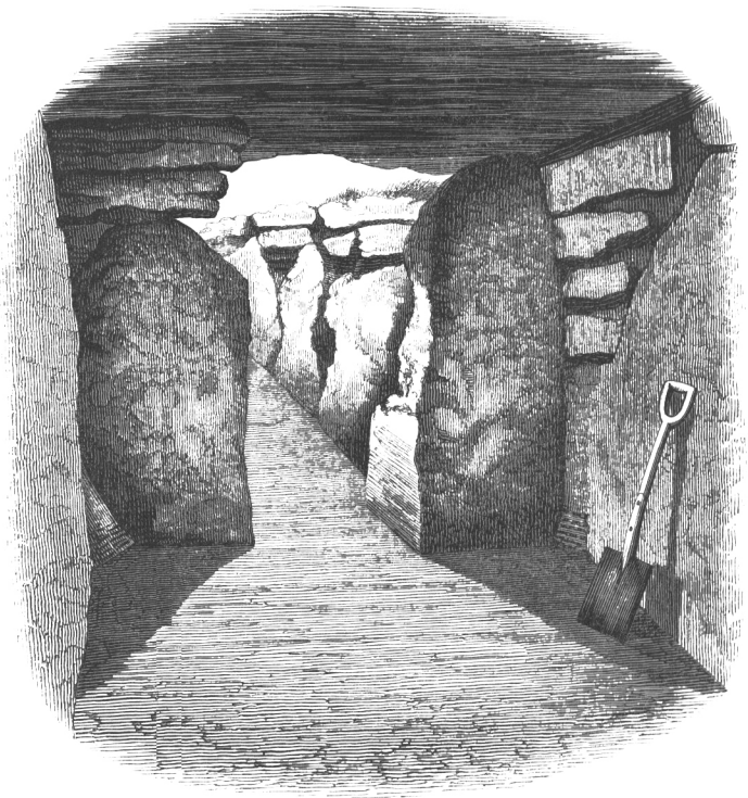
Fig. 6. View in the Chamber looking through the entrance.
