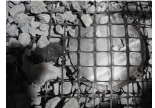
Placement of geogrid in the ballast layer
