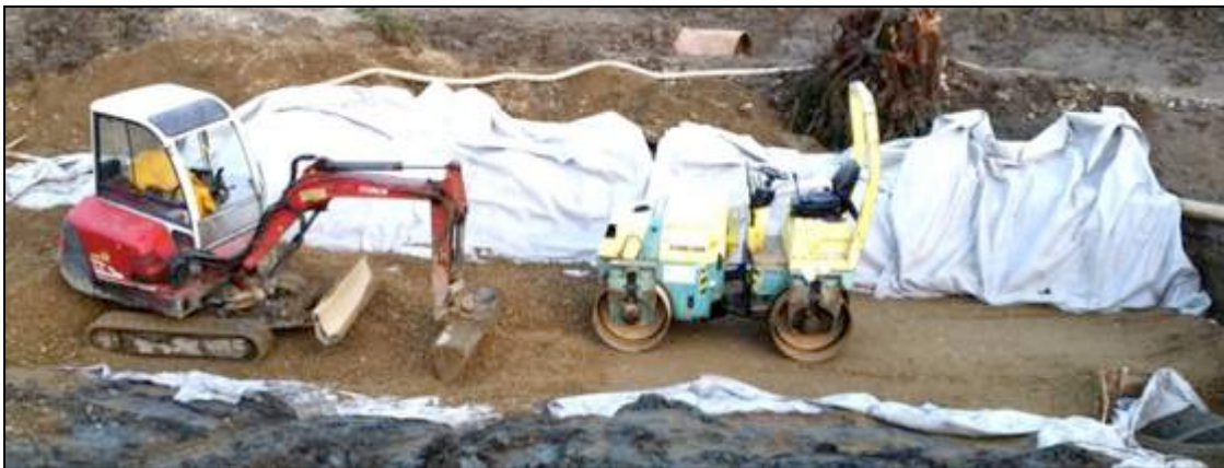
Construction of the gravel foundation, before wrapping the foundation with geosynthetics
