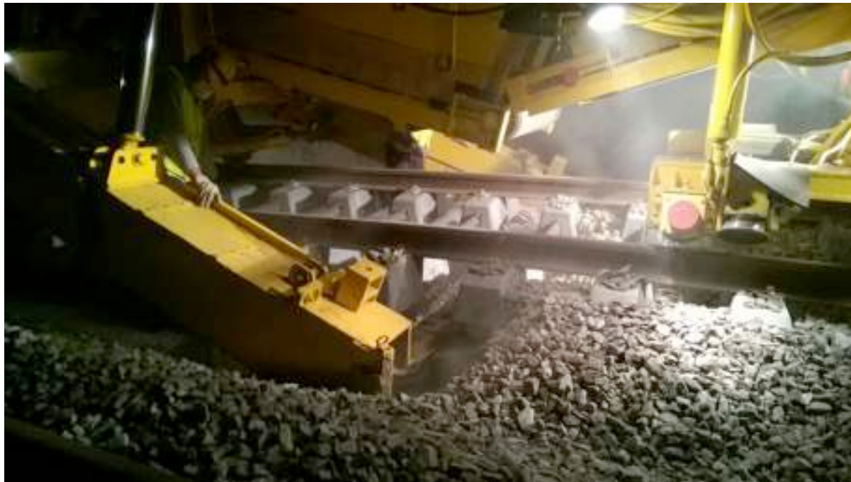
Track-mounted undercutting machine that rolls out the geogrid prior to new ballast being dropped in place over the geogrid
