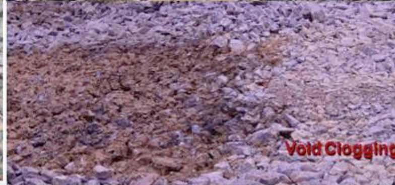
Subgrade Clay Pumping
