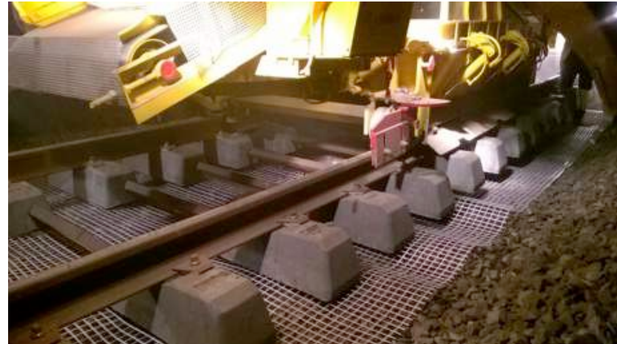
Track-mounted undercutting machine that rolls out the geogrid prior to new ballast being dropped in place over the geogrid
