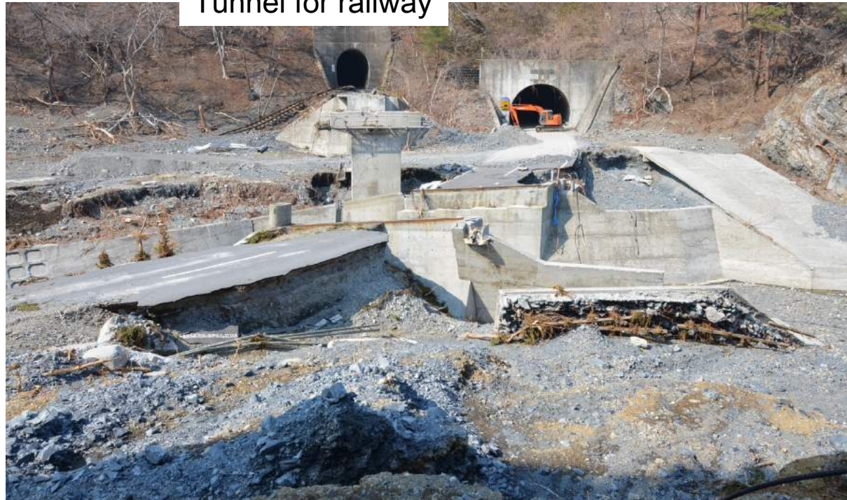
Tunnel for railway
