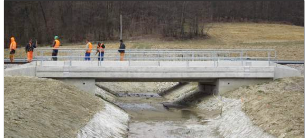
Conventional RC bridge with deep piled foundations
