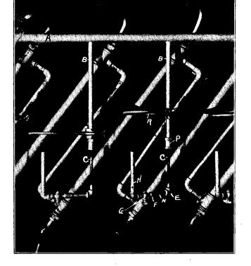
The gas pipe was already tapped for 1/8 in. air cocks to which the burners were attached. The air cocks were replaced by 1/8 in. close nipples. An II in. length of 9/16 in. (outside diam.) brass pipe, *B*, was tapped at one end to fit the 1/8 in. close nipple and
