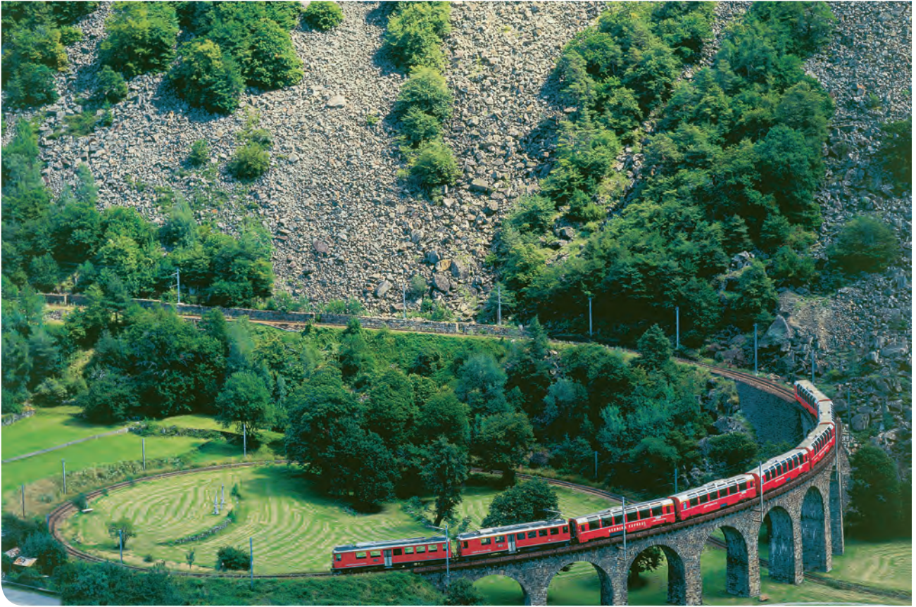
Photo 1: Circular viaduct of Rhaetian Railway near Brusio © Christof Sonderegger
