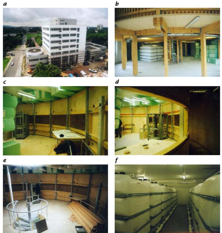
Fig. 2: a New building of the Institute for Environmental Physics in construction; b room below the facility; c to e interior of the annular wind/wave tunnel; f two rows of storage tanks, one for sea water and one for deionized water
