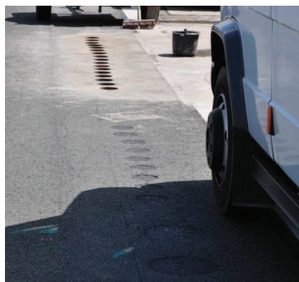
Fig. 1. Drilling core extraction on the test road tracks.
