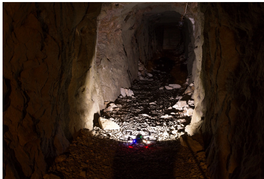
Fig. 1: Photo from an underground tunnel in Boden, Sweden for indicating the lighting conditions in a mine tunnel, while the effect of an artificial light source being also evident.
