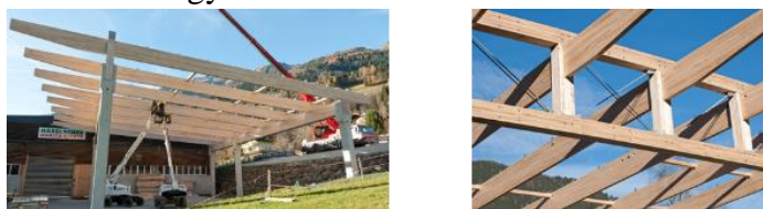
Figure 1: Pilot project in Carinthia made with birch GLT, industrial hall covering 1,000 m 2 with largest free span of 27 m and a maximum cross-section of the main girder of 100x1000 mm
