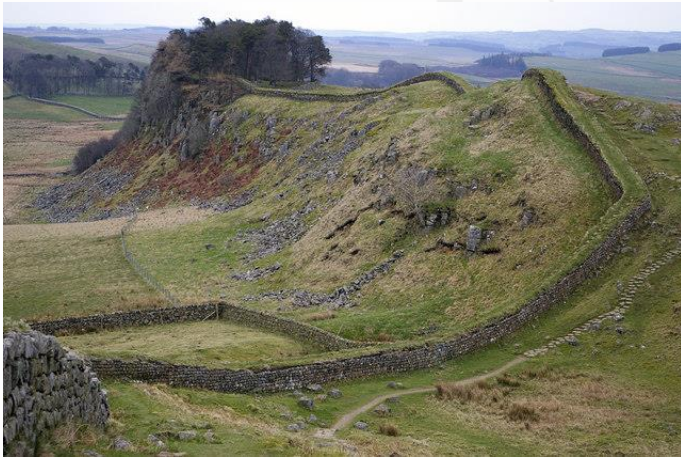
Phil Champion / Hadrian's wall at Cuddy's Crags and Housesteads Crags CC BY-SA 2.0 https://commons.wikimedia.org/wiki/File:Hadrian%27s_wall_at_Cuddy%27s_Crags_and_Housesteads_Crags_-_geograph.org.uk_-_404992.jpg
