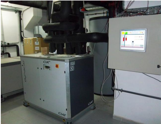
Figure 2: Ground-Med heat pump and local data logging system at Coimbra Regional Authority building
