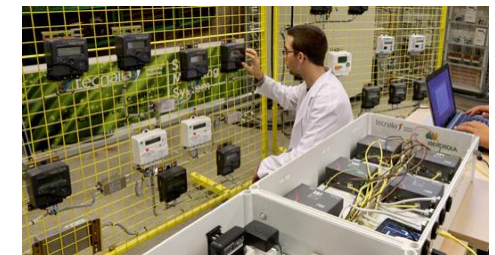
Smart metering communication platform at TECNALIA
