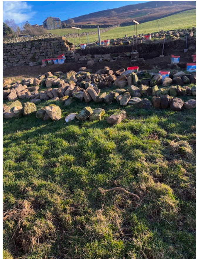
Fig. 7. Rebuilding a boundary wall in Danby Dale, North Yorkshire. October 2023.
