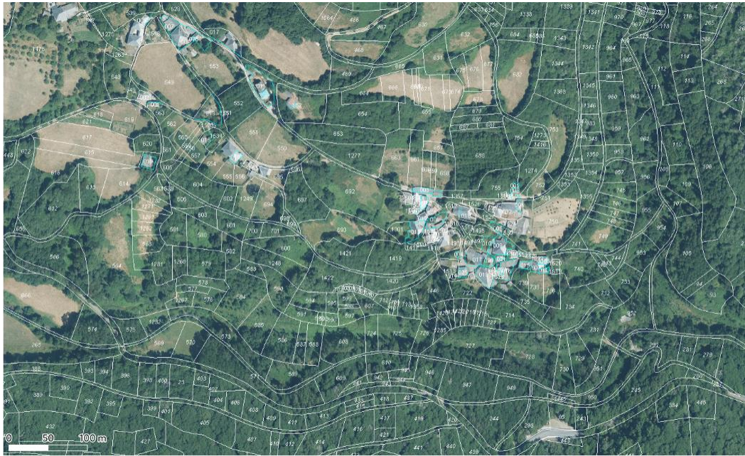
Figure 70 One of the currently declared model settlement projects. Note the proximity of forest and shrublands to the main group of houses in the middle of the image and the high levels of fragmentation.
