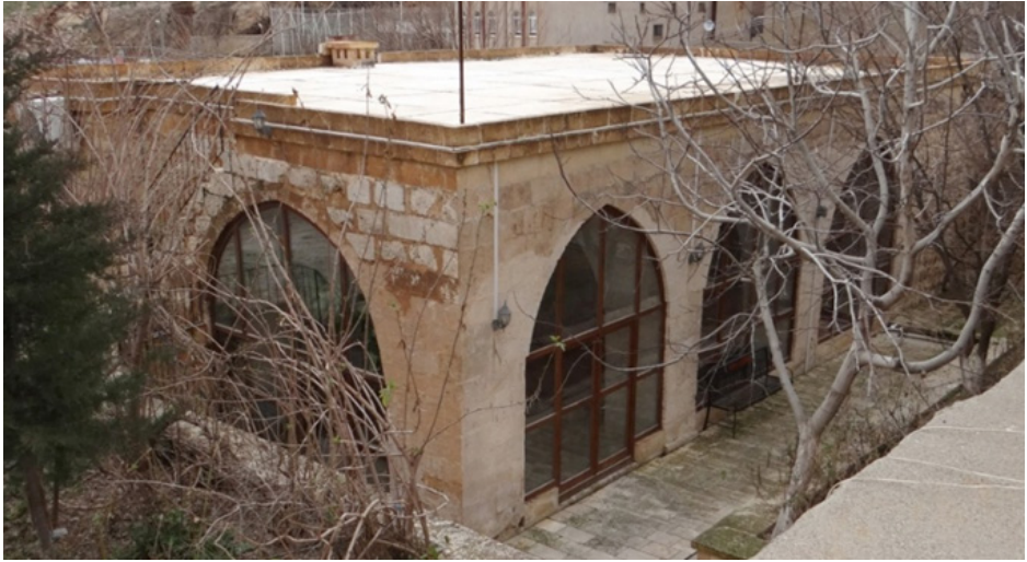
Figure 11: The masjid (view from northwest)
