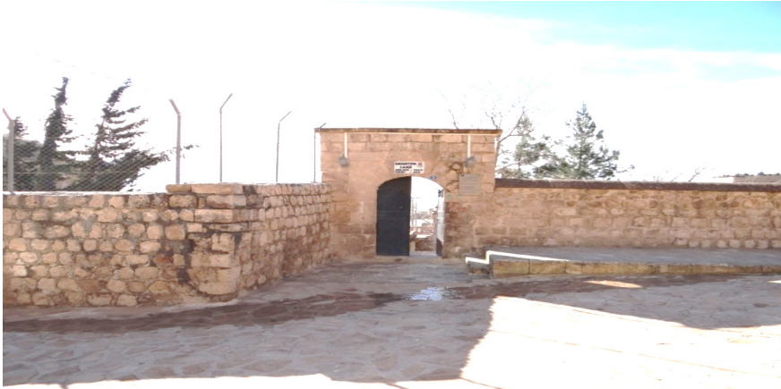
Figure 7: Main entrance of the complex (view from the north)
