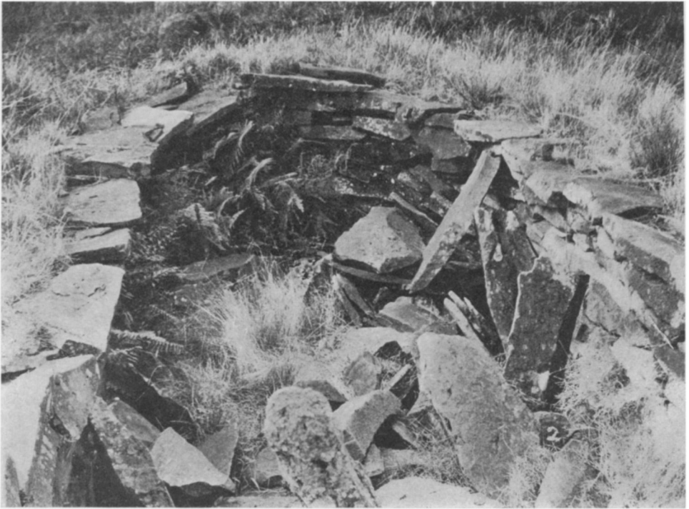
1. END OF A HOUSE UNROOFED. NO. 2.
