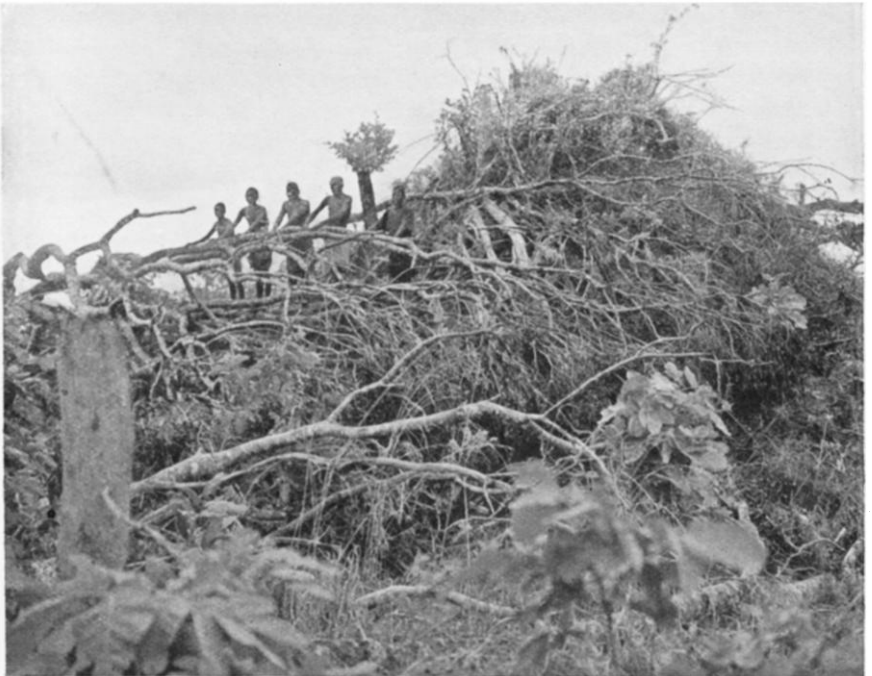
CLEARING AN AFRICAN AERODROME
