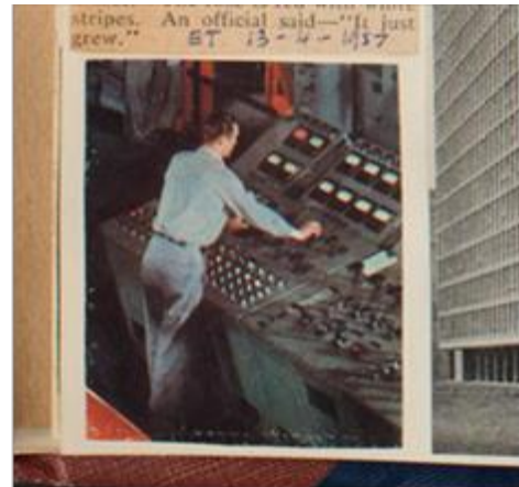
Image 15: Colour photograph of a man operating a control panel
