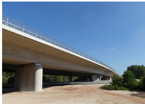
Fig. 3 Smart Bridge in the “Digital Test Area Autobahn”
