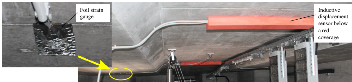
Fig. 5 Foil strain gauges and inductive displacement sensor on the bottom of the bridge deck slab (IBF)
