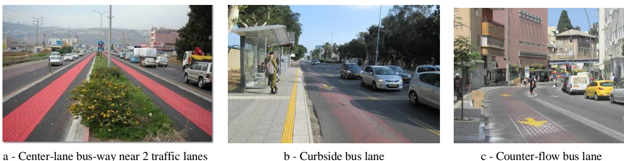
Fig. 2 Examples of bus lane configurations in Haifa BRT system
