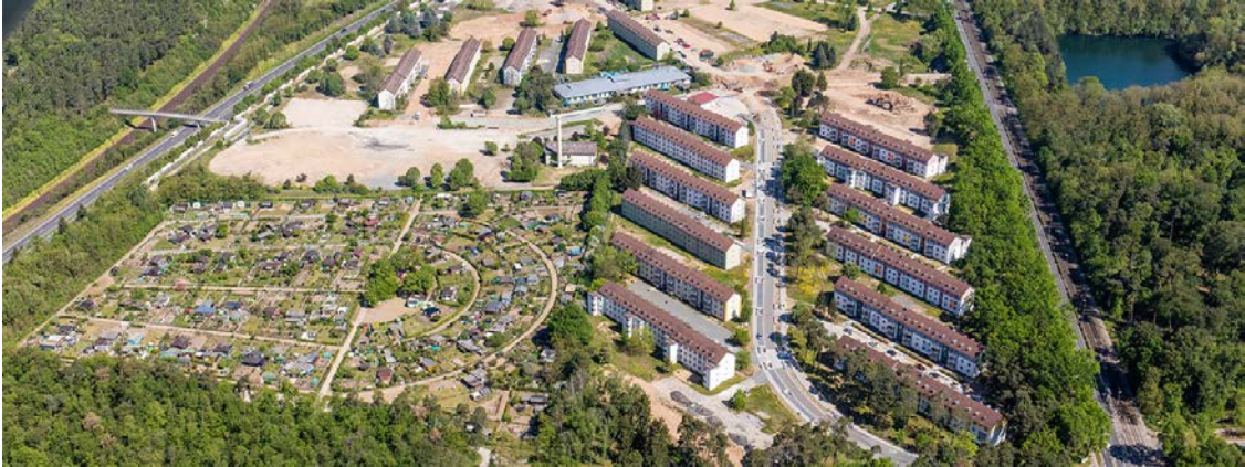
Fig. 2 Building construction in progress of the Lincoln-Siedlung in 2017
