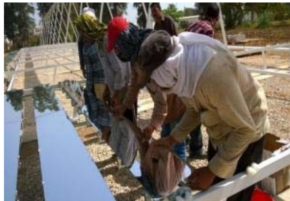
Figure 9. Installation works in the twinned plant in Egypt
