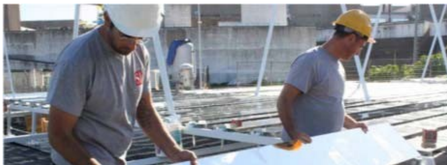
Figure 8. Local company staff at work in the demo plant
