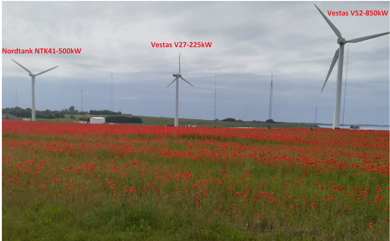
Figure 3.2: Risø test site in June 2019.
