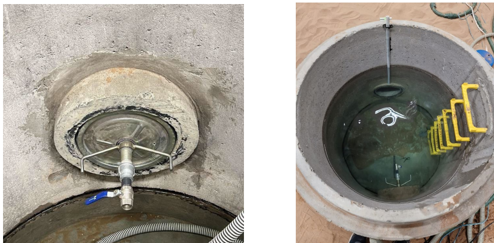
Figure 14. Manhole 4 (upstream) sealed; water level high at start of exfiltration test
