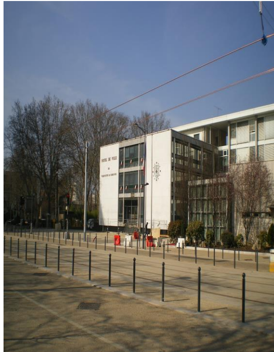
View of the town hall in Villeneuve-la-Garenne
