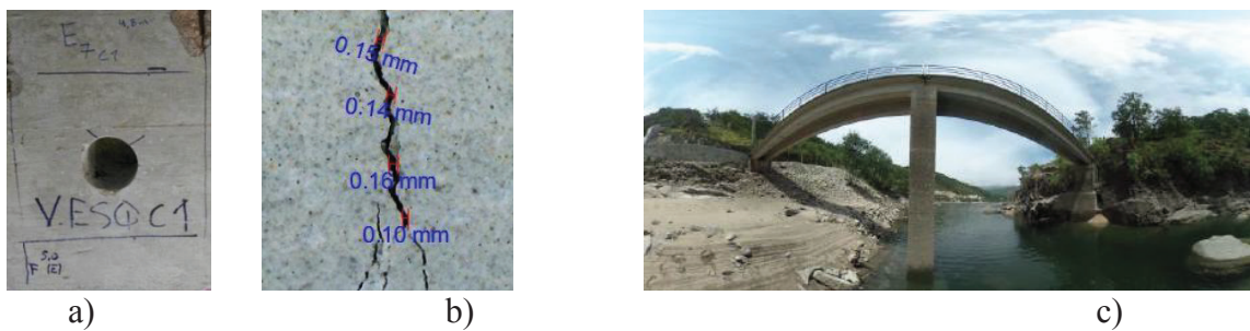
Figure 4: Inspection techniques: a) core extraction; b) crack width; c) 360° photography.
