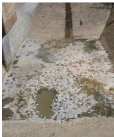
a) Abrasion in stilling basin
