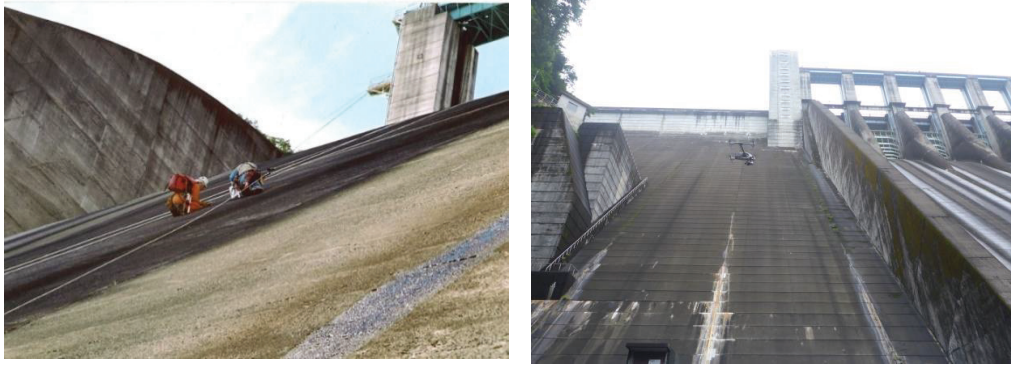
Figure 1: (Left photo) Climbing survey, (Right photo) UAV.
