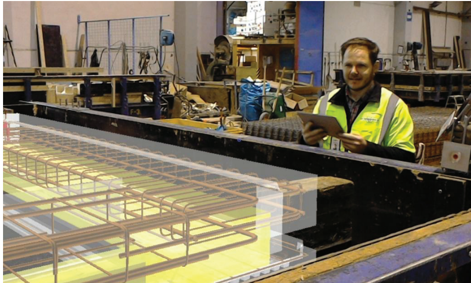
Figure 4: Digital element in the mould at SCF Betongelement AB factory in Strömsund Sweden picture from Information Experience.
