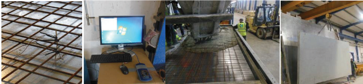
Figure 2: From left to right – Thermocouples attached on the reinforcement bars, temperature logging system, concrete wall casting on heating bed, wall lifted [photographs: F. Kanavaris].
