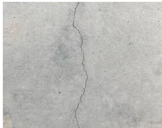
Figure 7: Surface cracking.
