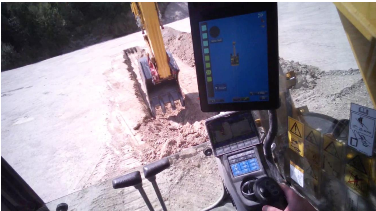
Figure 17: Excavator cabin view.
