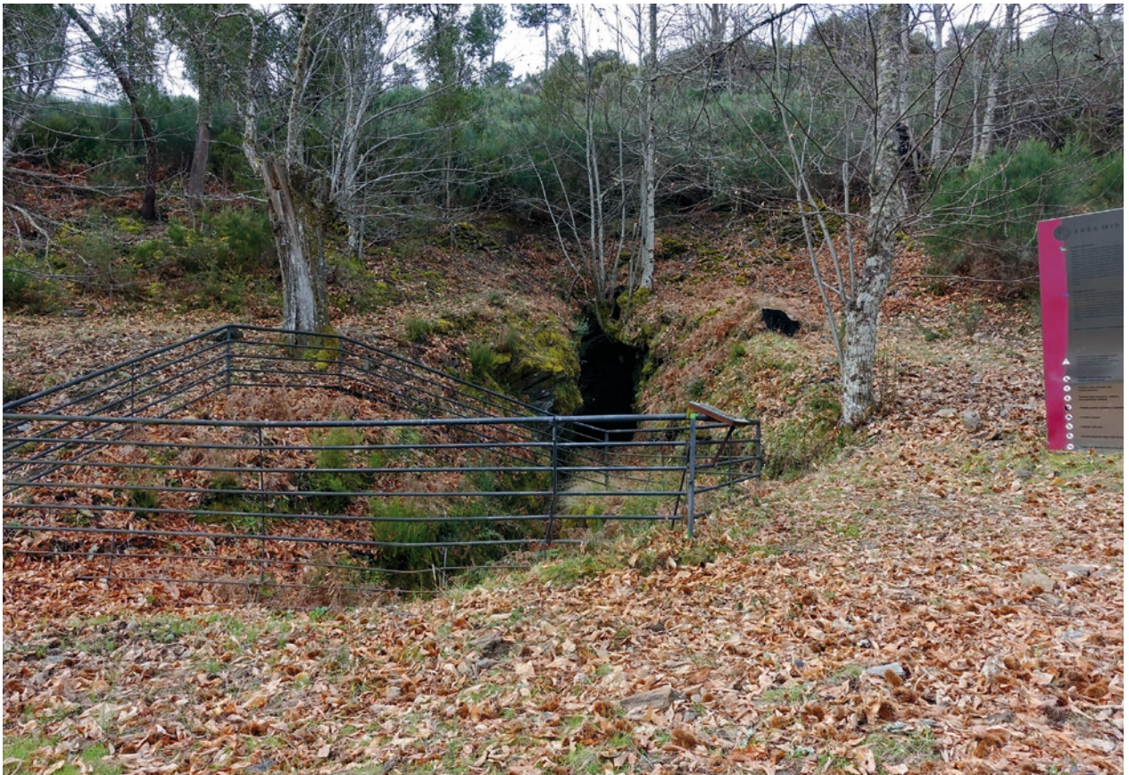
Fig. 3.3-15: Territorium metallorum Tresminas / Jales, Tresminas, Corta de Covas, Galeria do Pilar: the tunnel port area buried by the slope debris has only been partially exposed. The fence secures the connecting shaft to Galeria do Texugo (photo: R. Wahl-Clerici).
