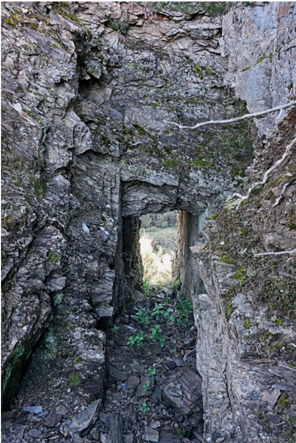
Fig. 3.0-7: Territorium metallorum Tresminas / Jales, Tresminas, Corta de Covas, from the south: view on the stairwell shaft for prospection (photo: R. Wahl-Clerici).
