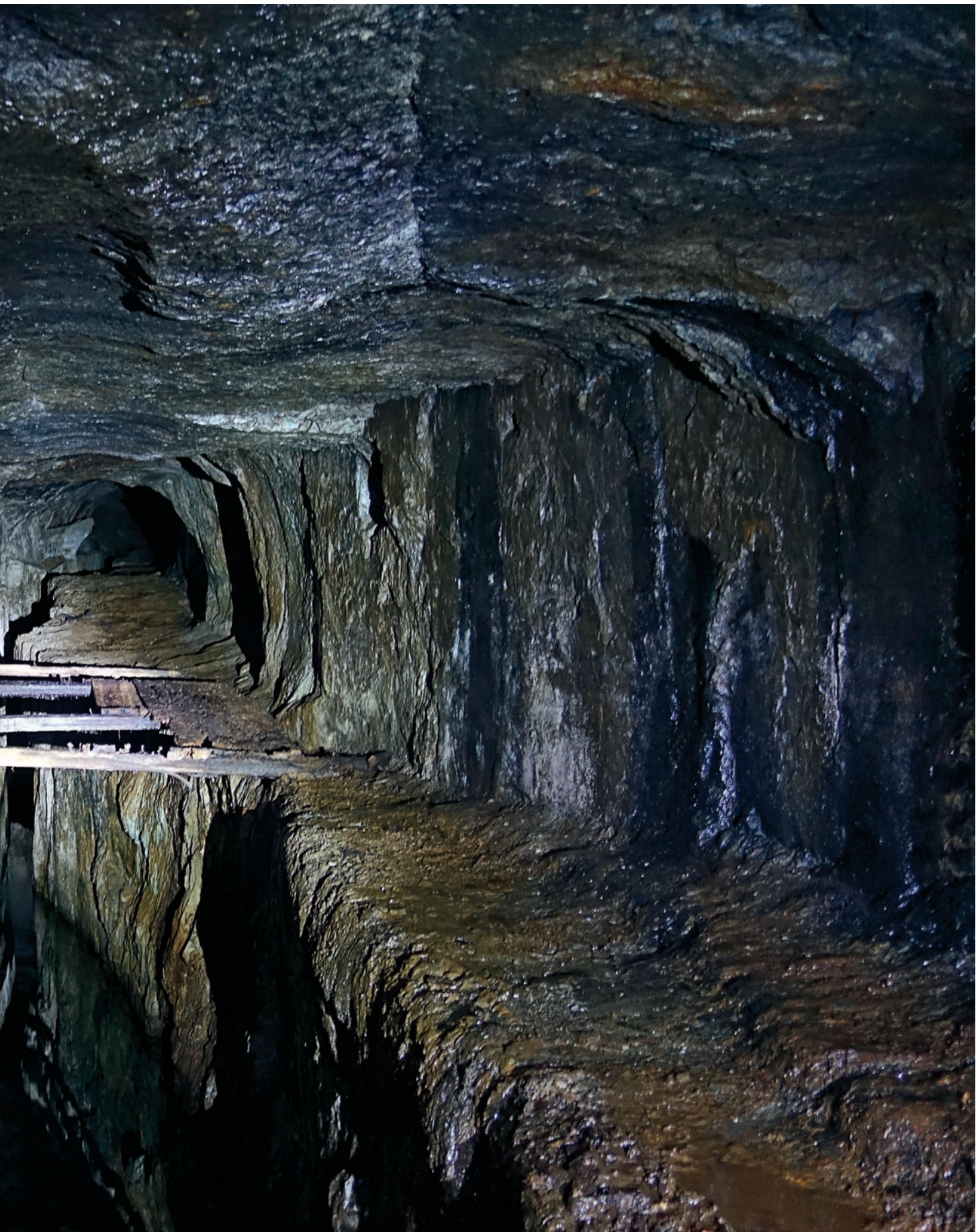
Fig. 3.3.1-5: Territorium metallorum Tresminas / Jales, Tresminas, Galeria do Pilar: collapse of the western side wall of the channel with the remains of a modern bridge to cross it. In the ceiling the first tunneling is still visible (photo: R. Wahl-Clerici).
