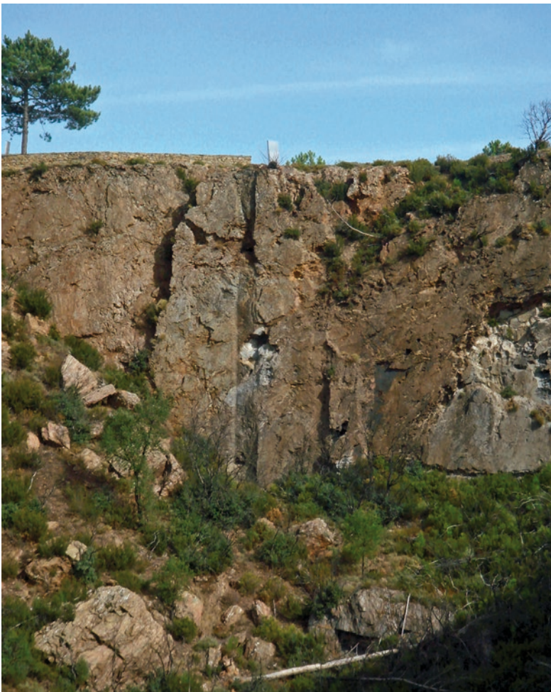
Fig. 3.0-11: Territorium metallorum Tresminas / Jales, Tresminas, Corta de Covas, from the west: eastern slope with the twin shafts, which were connected by galleries on several levels (photo: R. Wahl-Clerici).
