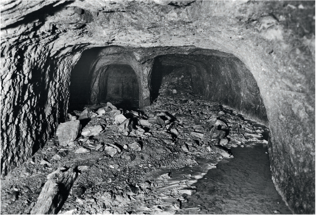
Fig. 3.3.1-15: Territorium metallorum Tresminas / Jales, Tresminas, Galeria do Texugo: change of the original course of the gallery in the area of the connecting shaft in the entrance area of the Galeria do Pilar (photo: J. Wahl).
