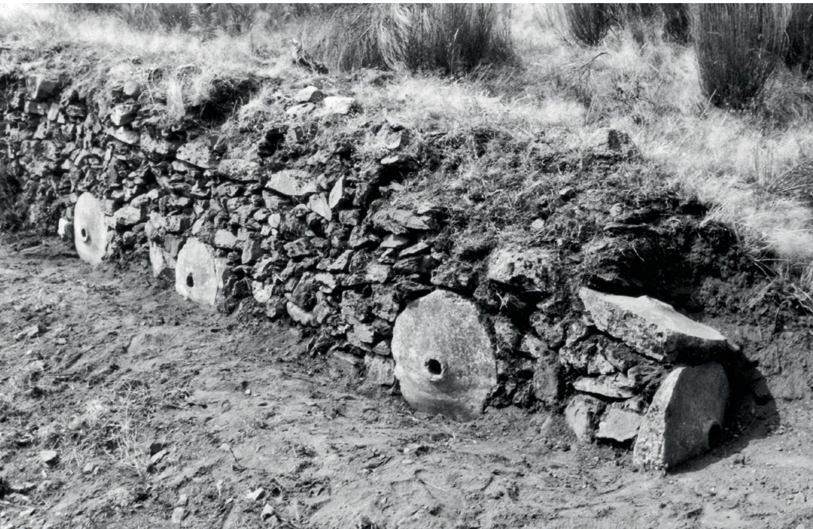
Fig. 4.0-23: Territorium metallorum Tresminas / Jales, Forno dos Mouros: modern wall built with millstones for ore crushing (photo: J. Wahl).
