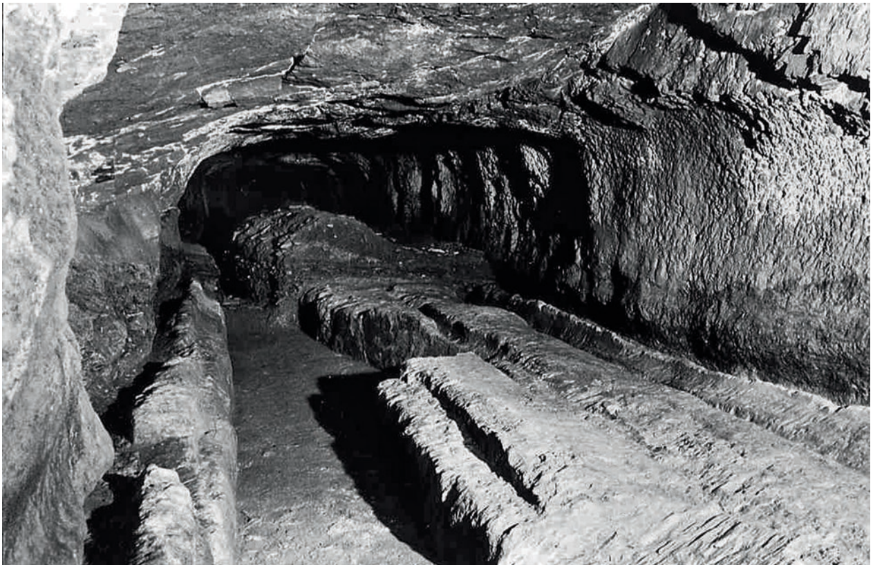
Fig. 3.3-2: Territorium metallorum Tresminas / Jales, Tresminas, Galeria do Pilar, seen from the north. The tunnel port area with cart tracks and drainage channel. The small older drainage channels are visible along the sides (photo: J. Wahl).
