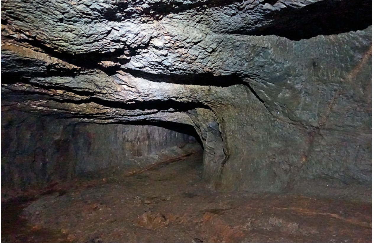
Fig. 3.3-30: Territorium metallorum Tresminas / Jales, Tresminas, Corta da Ribeirinha, Galeria dos Morcegos: zone in the area of the first change of direction from the tunnel port with target width of 3.85 m. The former working faces of the tunnel and the cuts between them are clearly visible in the roof (photo: R. Wahl-Clerici).
