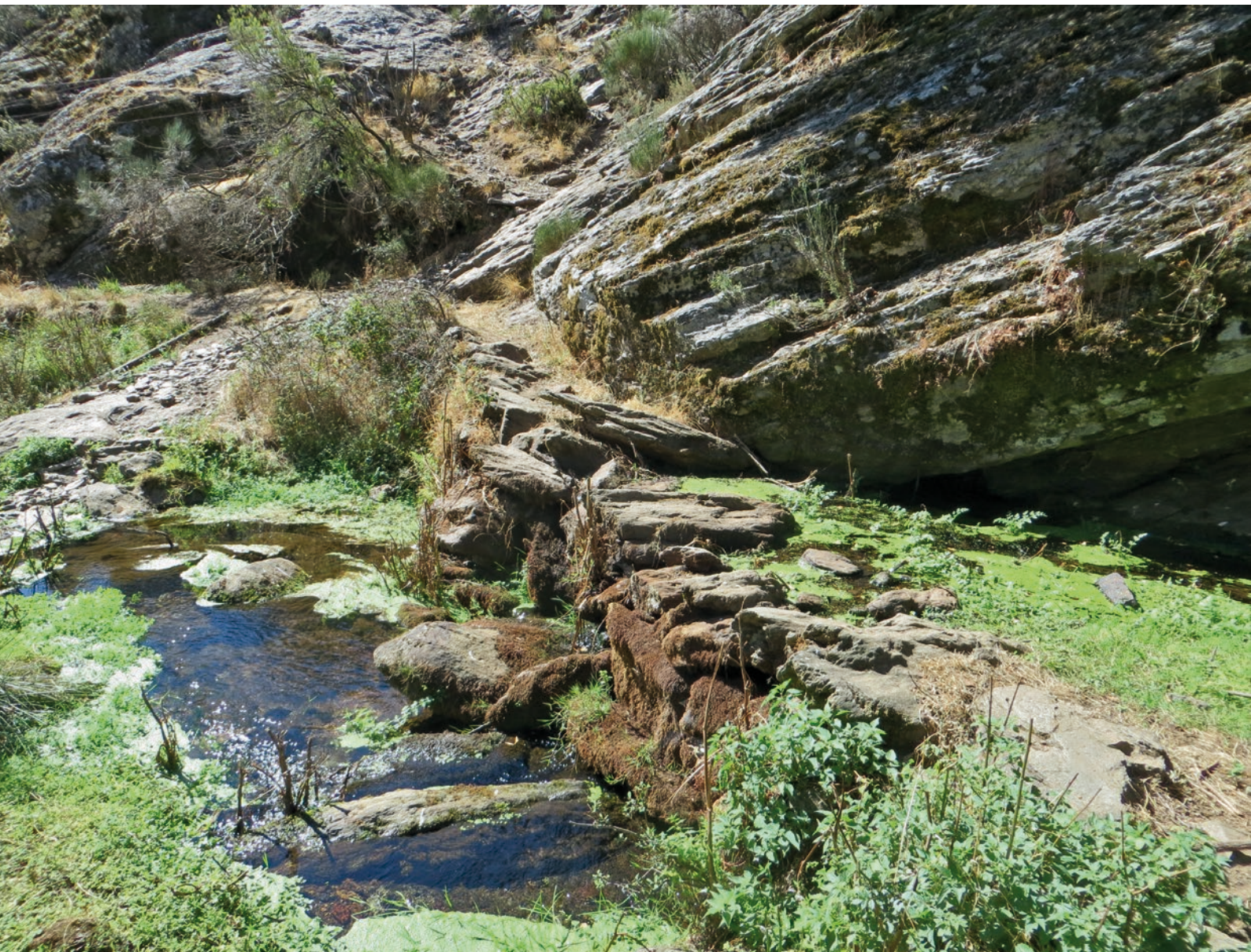
Fig. 5.0-20: Territorium metallorum Tresminas / Jales: Sevivas weir, the C4 aqueduct to the mining zone of Tresminas was fed from here. The cuts in the large rock mark the beginning of the channel (photo: R. Wahl-Clerici).
