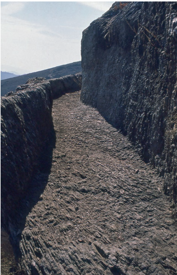
Fig. 5.0-35a/b: Territorium metallorum Tresminas/Jales, Sevilas, Vale do Ribeiro do Cão: part of channel C2 was completely cut into the rock. Well preserved are the carvings in the rock made to position the stones of the accompanying wall (photos: J. Wahl).
