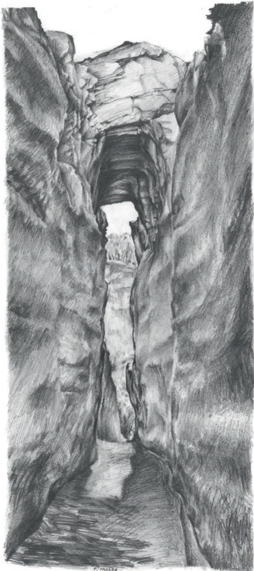
Fig. 3.0-22: Territorium metallorum Tresminas / Jales, Tresminas, Corta da Ribeirinha: the upper level of the prospecting system at the western entrance. The oldest carefully worked trapezoidal gallery is still well visible, they were sunk in stages (drawing: P. Moser).
