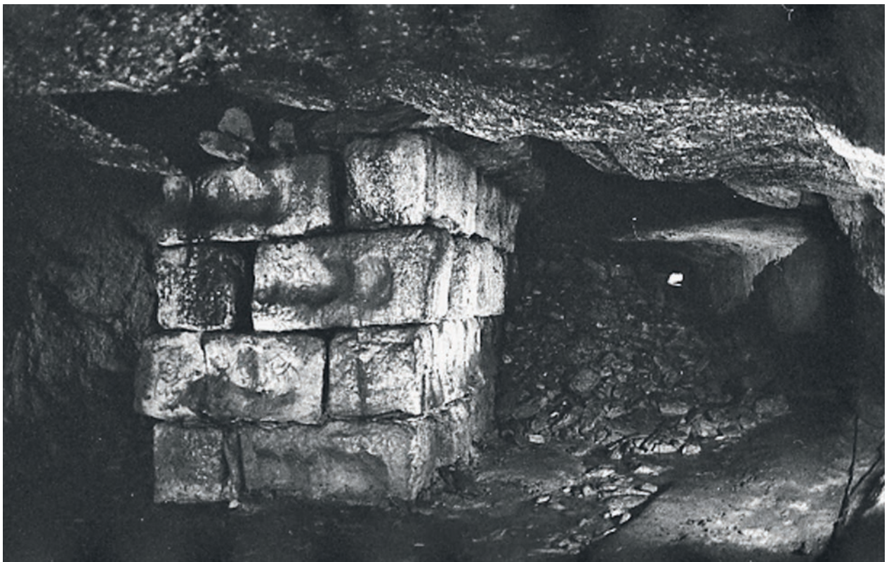
Fig. 3.3-17: Territorium metallorum Tresminas / Jales, Tresminas, Corta de Covas, Galeria do Pilar, seen from the south: to the left of the picture the eponymous pillar, and to the right the extension for the passage of transport and the drainage channel. The tunnel port is visible in the background as a bright spot (photo: C. Wahl).
