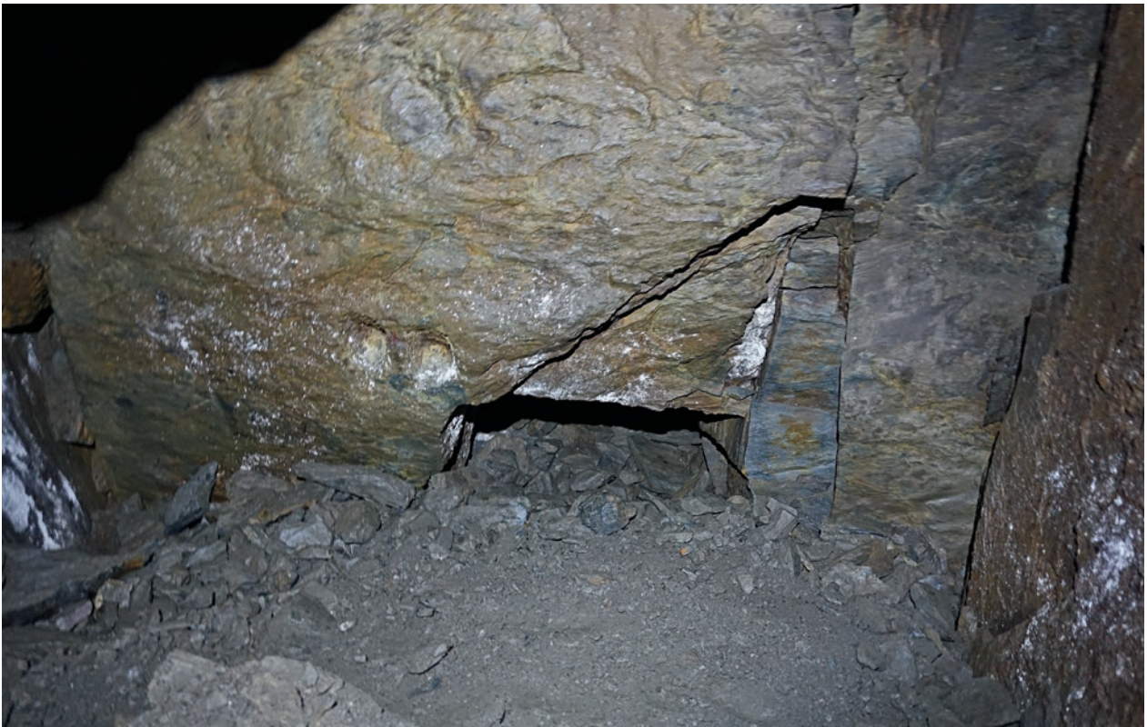
Fig. 2.1-7: Territorium metallorum Tresminas / Jales, Tresminas, Galeria dos Alargamentos: view of the collapsed roof of the stairwell at position D. Two of the three cuts in block 2 can be seen (photo: R. Wahl-Clerici).
