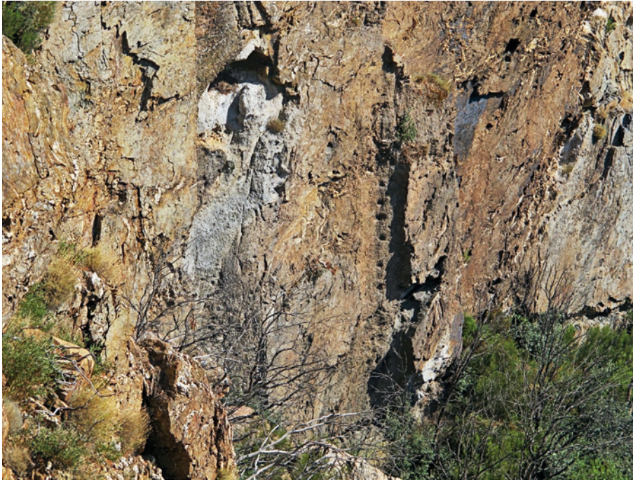
Fig. 3.3-9: Territorium metallorum Tresminas / Jales, Tresminas, Corta de Covas: eastern slope with the twin shafts, which were inside the mountain in Roman times. To the right: riser shaft with the cuts for the risers, to the left: winding shaft. The latter pierces the end chamber of Galeria dos Alargamentos (photo: R. Wahl-Clerici).
