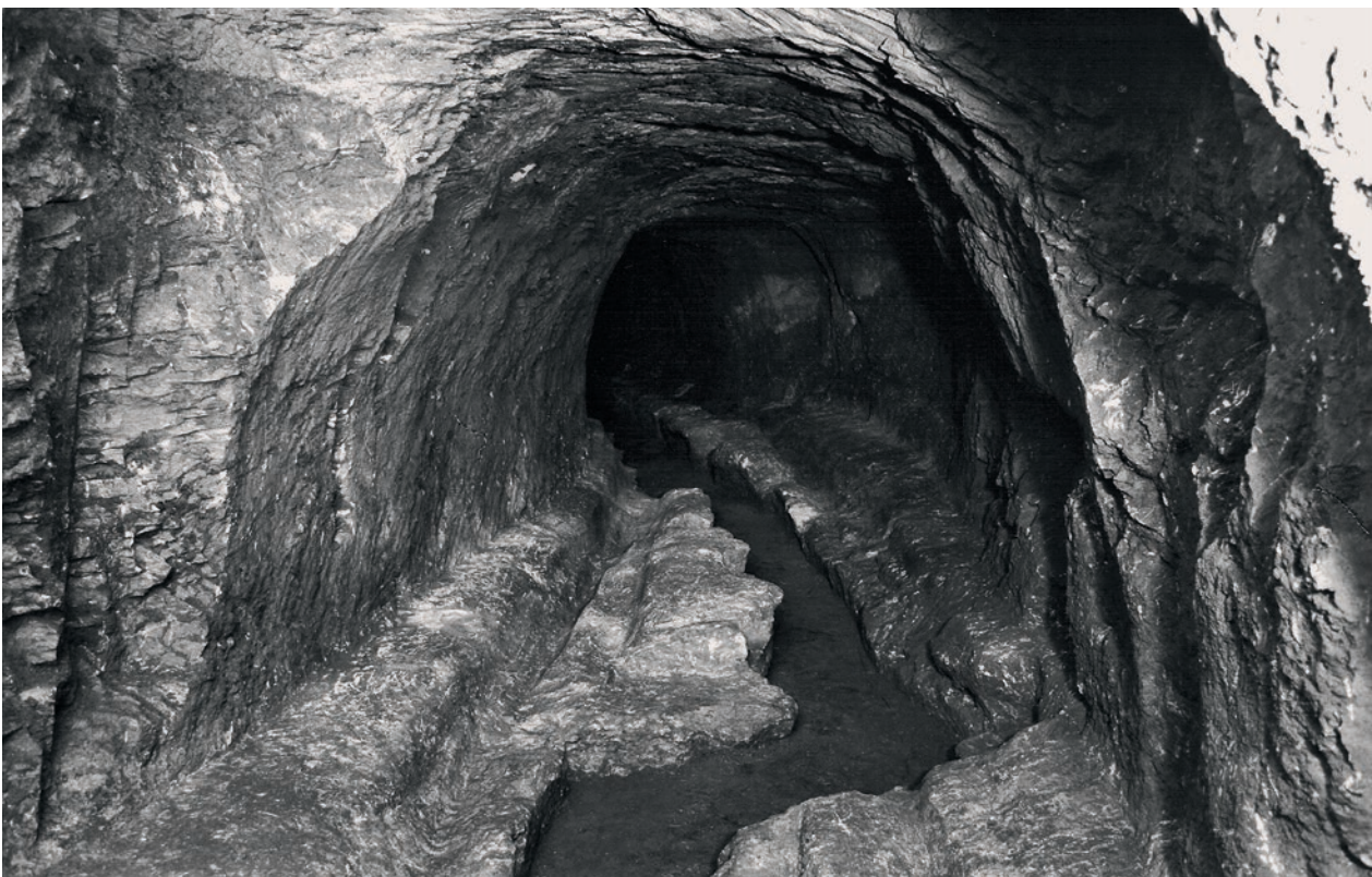
Fig. 3.3.1-7: Territorium metallorum Tresminas / Jales. Tresminas, Galeria Esteves Pinto: the cross section is close to the form of a segment of a circle, entrance area from the outside (photo: J. Wahl).
