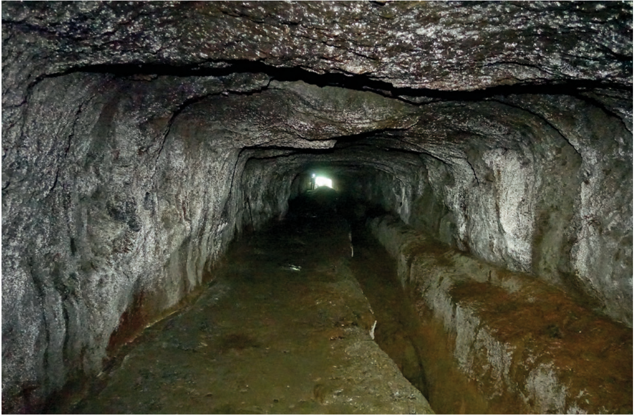
Fig. 5.0-36: Territorium metallorum Tresminas / Jales, Tresminas, Galeria do Pilar, from the south: drainage channel on the eastern working face (photo: R. Wahl-Clerici).
