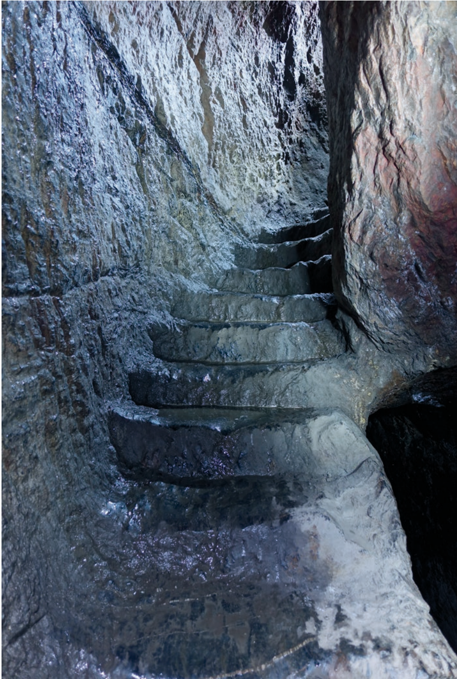
Fig. 2.2-13: Serra da Santa Justa, Valongo (conc. Valongo, distr. Porto), Fojo das Pombas: circular U-shaped staircase shaft, the staircase was continued straight after the lower section (photo: R. Wahl-Clerici).
