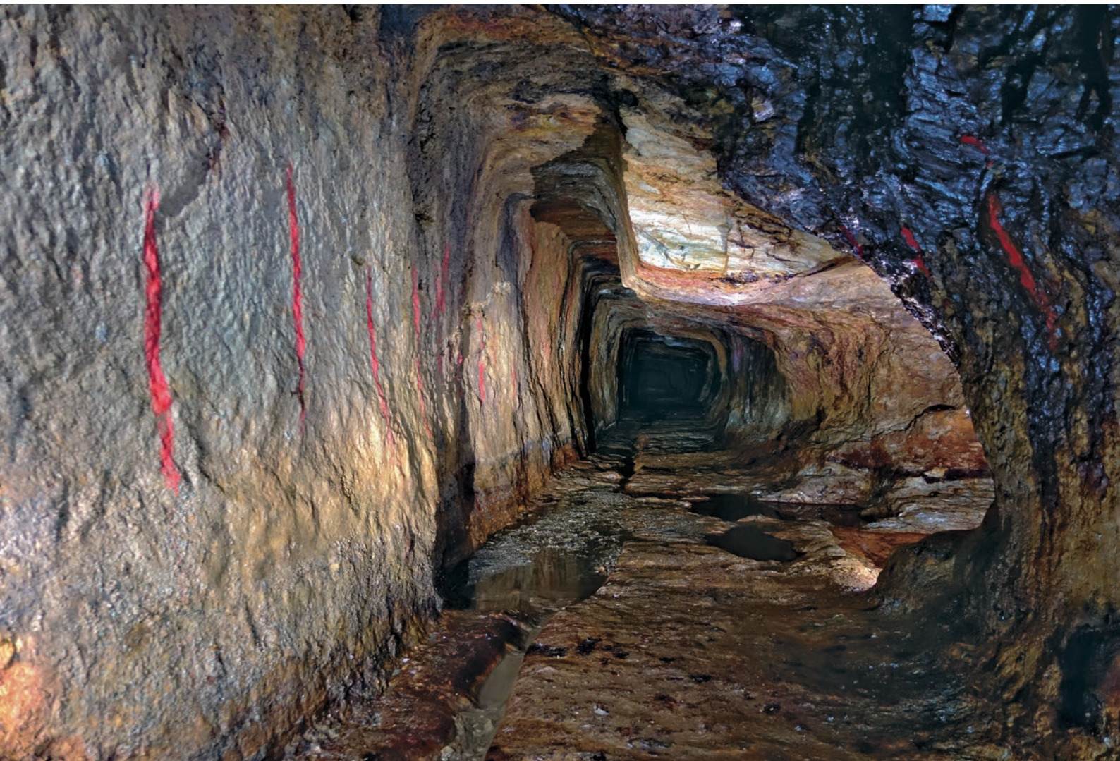
Fig. 3.3.1-18: Territorium metallorum Tresminas / Jales, Tresminas, Galeria dos Morcegos, from the south: the tunnel had to be lowered in some places by up to 80 cm. A slight extension was driven into the western working face in the area of the prospecting shaft (photo: R. Wahl-Clerici).
