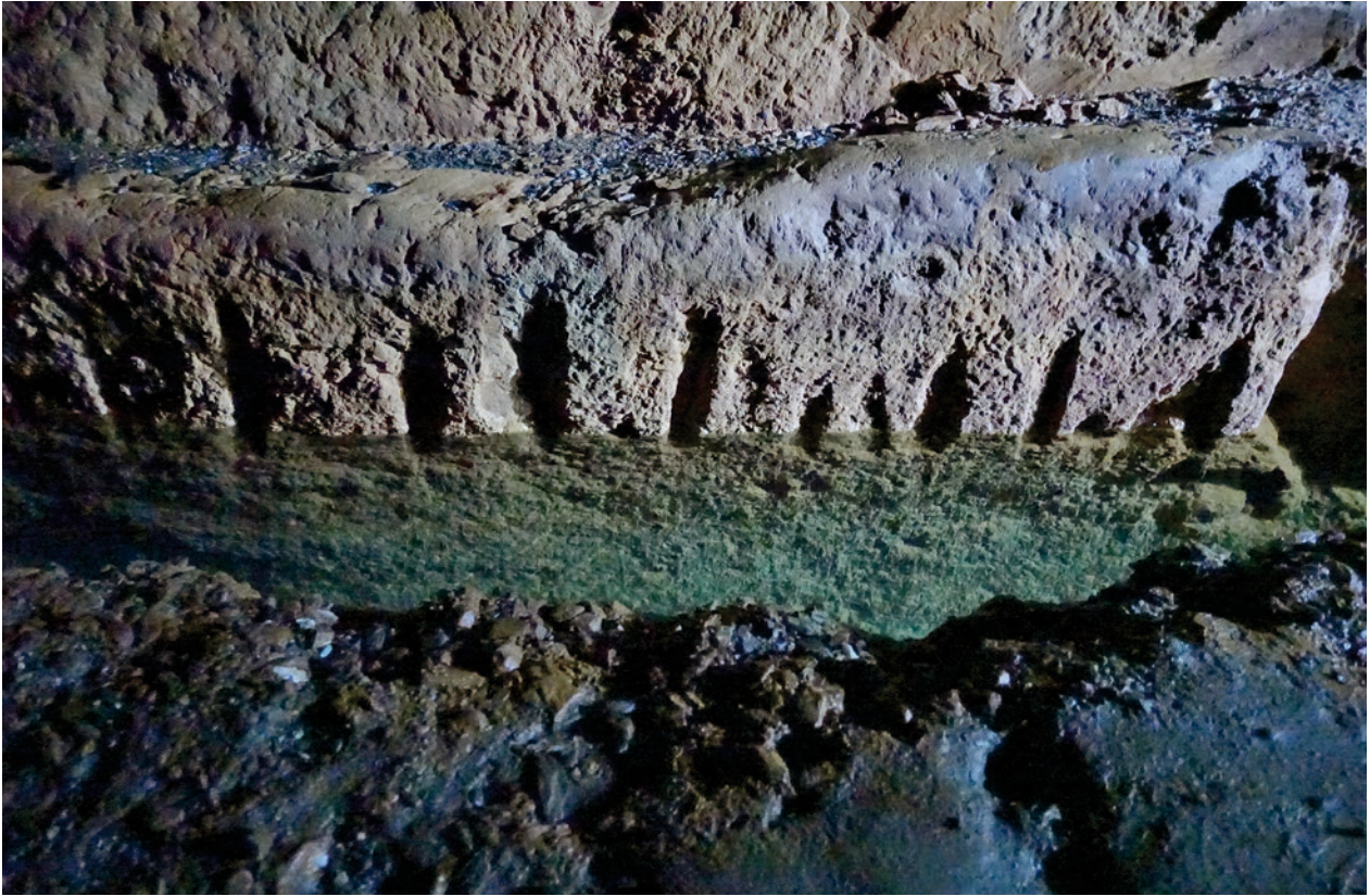
Fig. 3.3-18: Territorium metallorum Tresminas / Jales, Tresminas, Corta de Covas, Galeria do Pilar: cuts made for the wooden cover of the drainage channel (photo: R. Wahl-Clerici).
