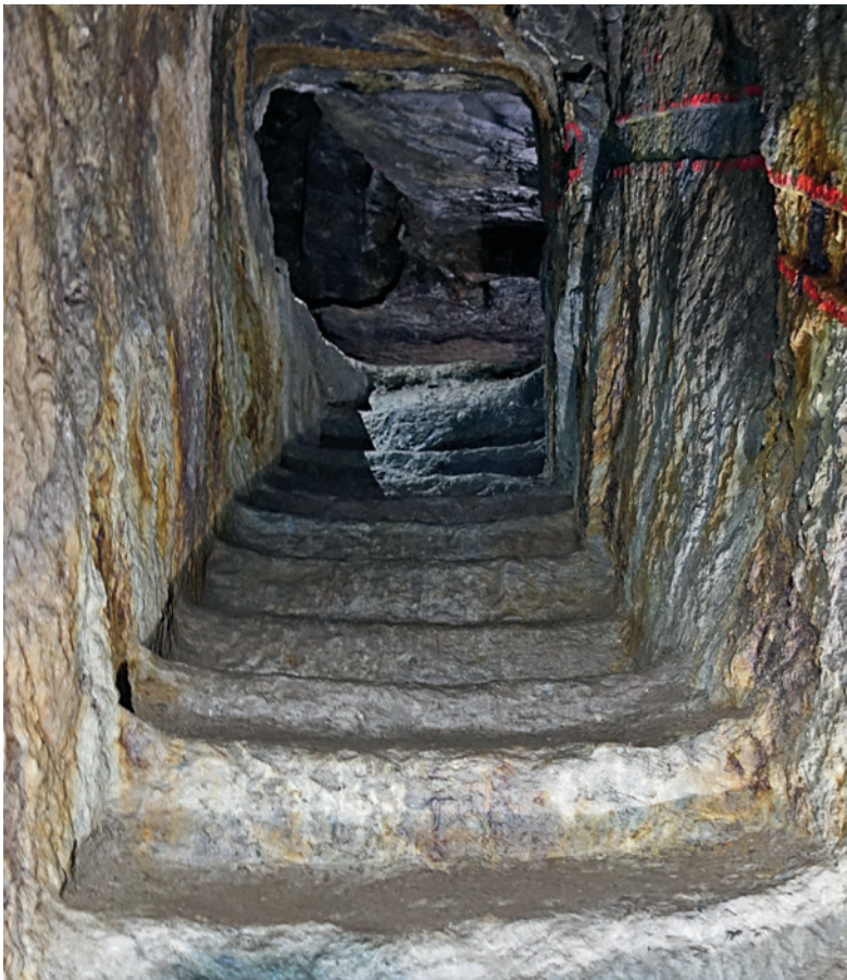
Fig. 2.1-3b: Territorium metallorum Tresminas / Jales, Tresminas, Galeria dos Alargamentos. View into the stairwell from the south (photo: R. Wahl-Clerici).
