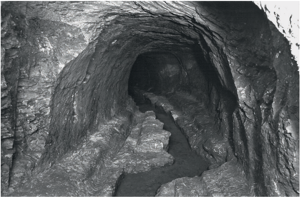
Fig. 3.0-8: Territorium metallorum Tresminas / Jales, Tresminas, Corta de Covas, from the south: entrance of the Galeria Esteves Pinto, with the drainage channel and cart tracks sunk into the sole (photo: J. Wahl).
