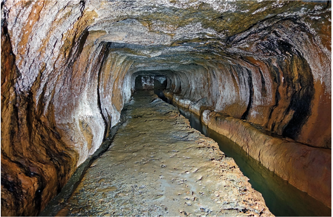
Fig. 3.3.1-3: Territorium metallorum Tresminas / Jales, Tresminas, Galeria do Pilar: situation behind the pillar. The conspicuous irregularity of the sides was caused by the working faces, which were driven into the rock to widen the cavity. View towards the entrance on the slope (photo: R. Wahl-Clerici).
