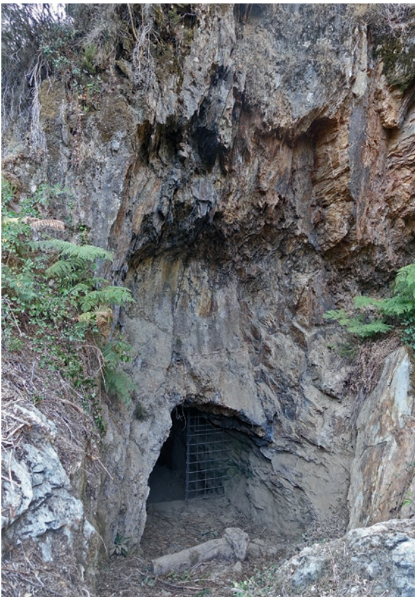
Fig. 2.2-9: Territorium metallorum Tresminas / Jales. Tresminas, Corta da Ribeirinha, Galeria do Pastor: the traces of hewing above the port bearing witness to the mining progress are clearly visible. This zone of the Galeria was once used for mining, while the lower areas of the Galeria consisted only of a gallery for prospecting. Seen from the southeast (photo: R. Wahl Clerici).
