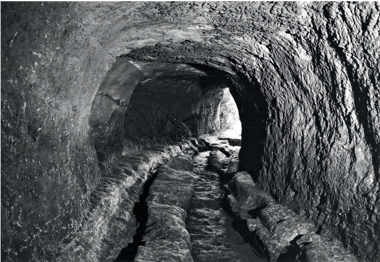
Fig. 3.3-13: Territorium metallorum Tresminas / Jales, Tresminas, Corta de Covas, Galeria Esteves Pinto: on the right side of the picture is the sighting shaft, with the cuts to cover the canal visible. View towards the tunnel port on the slope (photo: J. Wahl).
