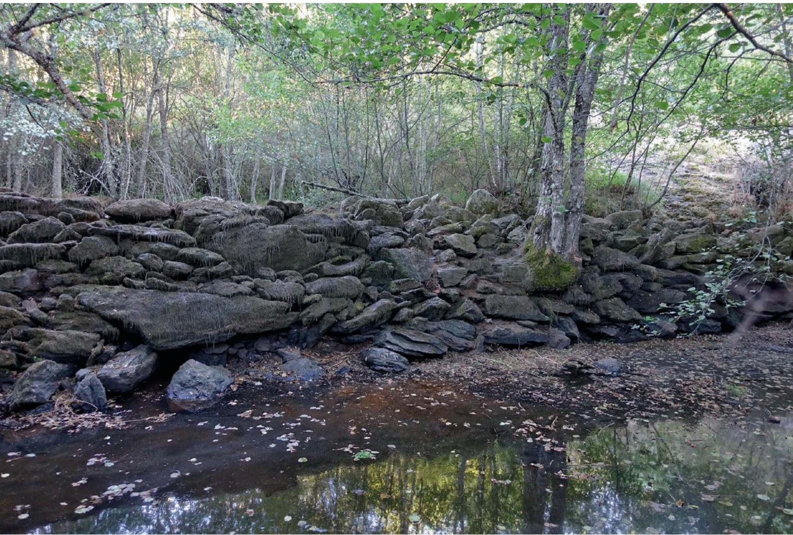
Fig. 5.0-22: Territorium metallorum Tresminas / Jales: weir of the Rio Tinhela in the Vale Curtinha. View from the valley, from the west. The bottom outlet is hidden under the large transverse boulder (photo: R. Wahl-Clerici).
