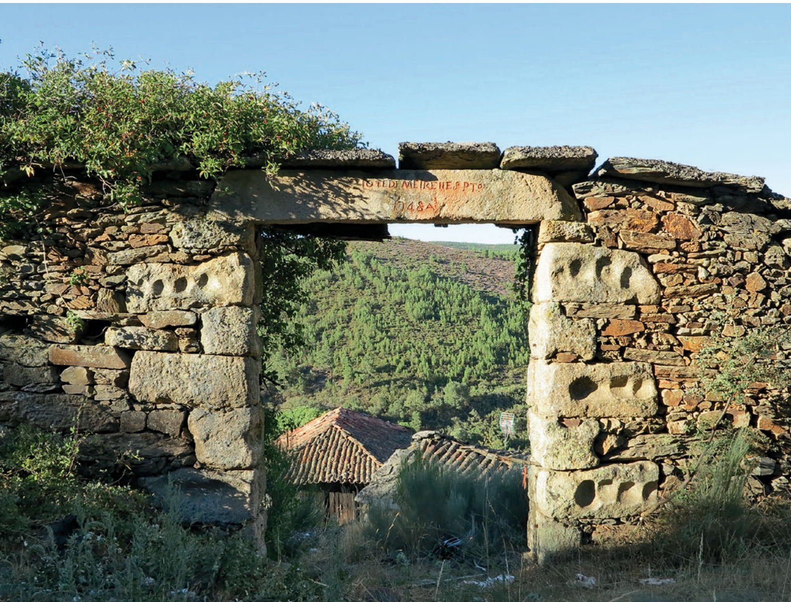
Fig. 4.0-14: Territorium metallorum Tresminas / Jales, Ribeirinha: arch made from the reused mortars (photo: R. Wahl-Clerici).
