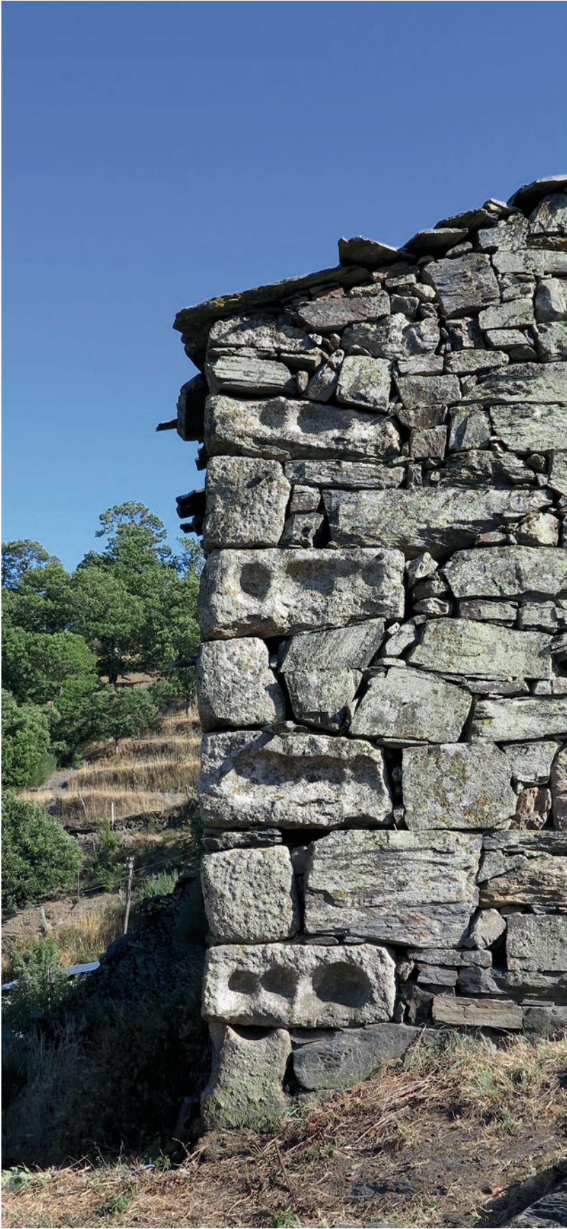
Fig. 4.0-9: Territorium metallorum Tresminas/Jales, Ribeirinha: use of the stamp mill bases from the extraction zone mostly as corner stones (photo: R. Wahl-Clerici).
