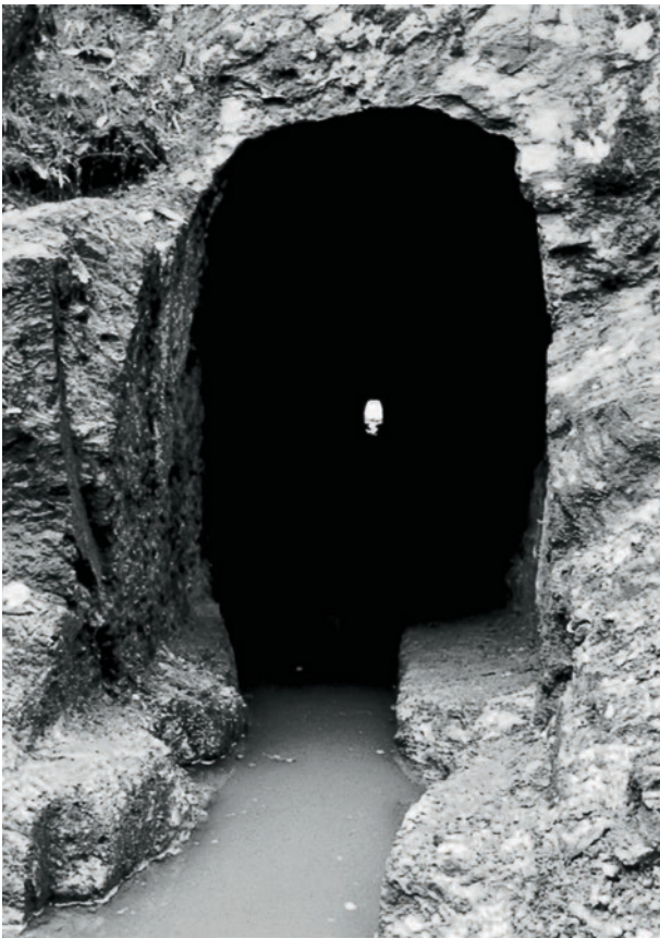
3.3-8: Territorium metallorum Tresminas / Jales, Tresminas, Corta da Ribeirinha, Galeria do Buraco Seco: tunnel port in the open pit mine (photo: J. Wahl).
