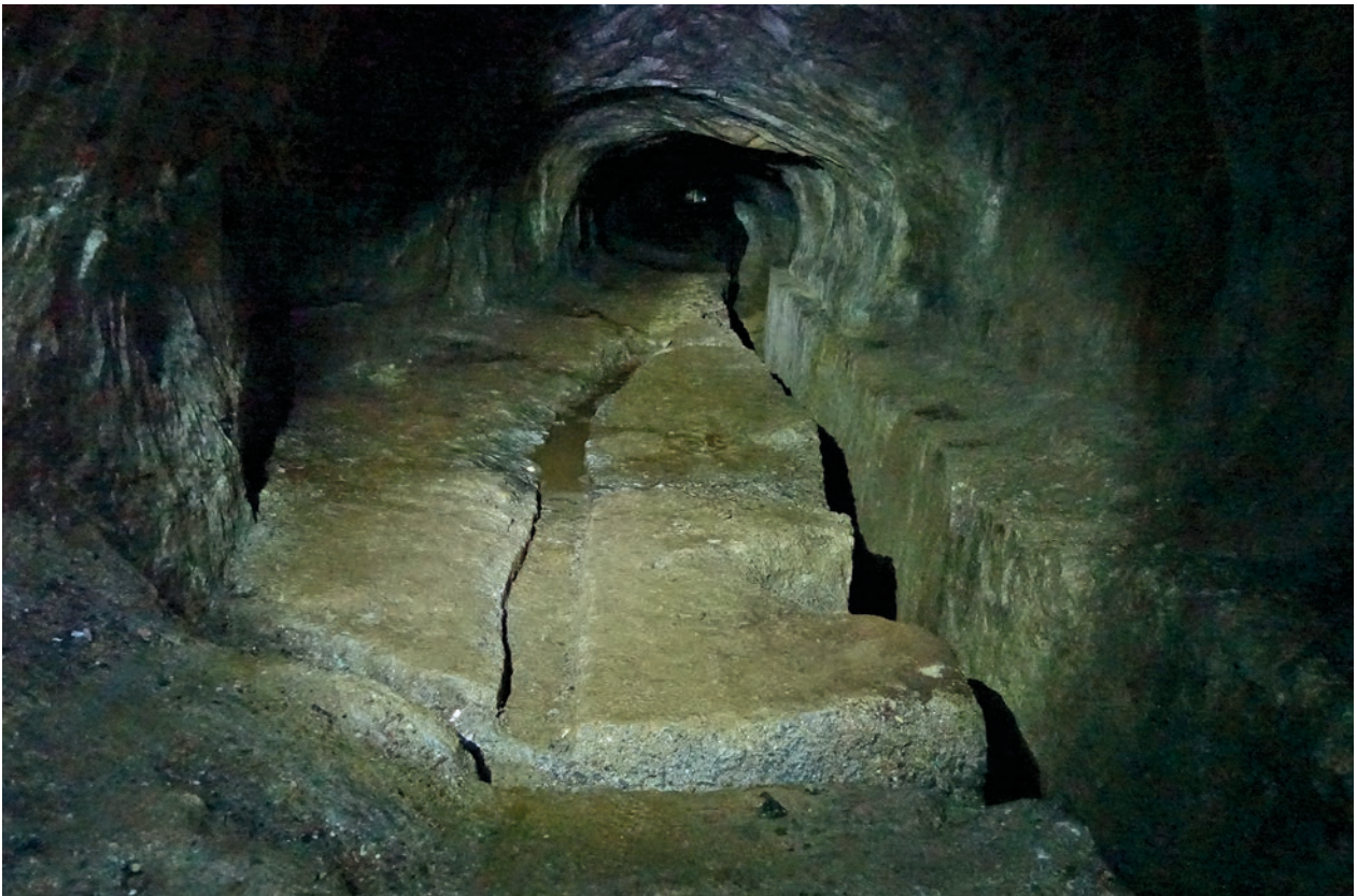
Fig.3.3-22: Territorium metallorum Tresminas / Jales, Tresminas, Corta de Covas, Galeria do Pilar: view from the south onto the narrow ditches that were first cut into the floor in order to lower the whole floor (photo: R. Wahl-Clerici).
