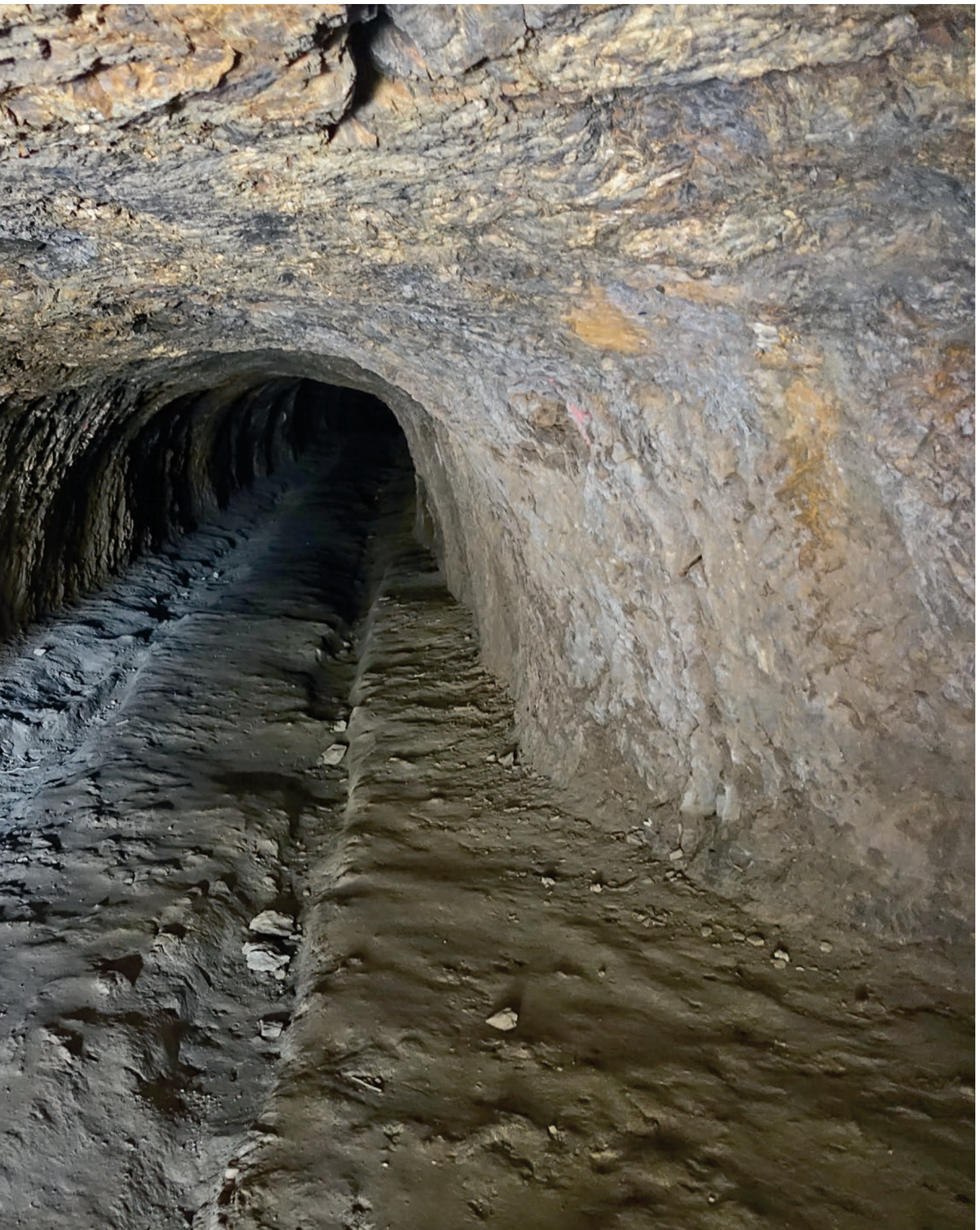
Fig. 3.3-11: Territorium metallorum Tresminas / Jales, Tresminas: the Galeria dos Alargamentos with one of the extensions to the right. The cart tracks in the floor do not touch any of the four extensions (photo: R. Wahl-Clerici).
