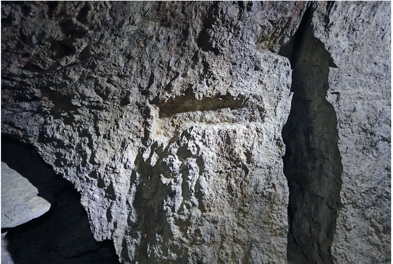
Fig. 2.1-8: Territorium metallorum Tresminas / Jales, Tresminas, Galeria dos Alargamentos: cuts in the rock in order to allow the insertion and securing of a crossbeam, in order to attach a winch to help with the clearing of debris during the rescue work (photo: R. Wahl-Clerici).
