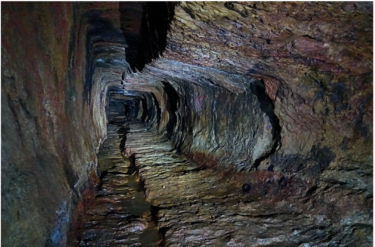
Fig. 3.3.1-4: Territorium metallorum Tresminas / Jales, Tresminas, Corta da Ribeirinha, Galeria dos Morcegos: part of the tunnel below the open pit mine; after lowering the first tunnel (on the left), the adit was enlarged towards the east (photo: R. Wahl-Clerici).
