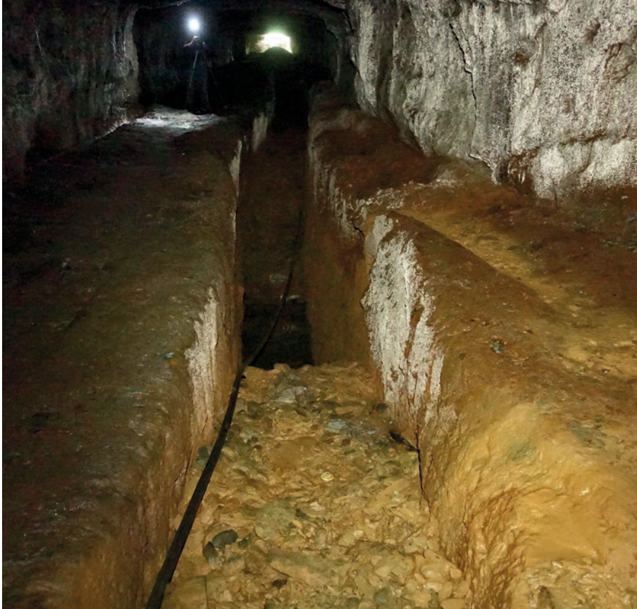
Fig. 3.2-20a/b: Territorium metallorum Tresminas / Jales, Tresminas, Corta de Covas, Galeria do Pilar: intentionally filled-up zone between the entrance and the blind shaft between the Galeria do Pilar and the Galeria do Texugo [FU11] (photo: R. Wahl-Clerici).
