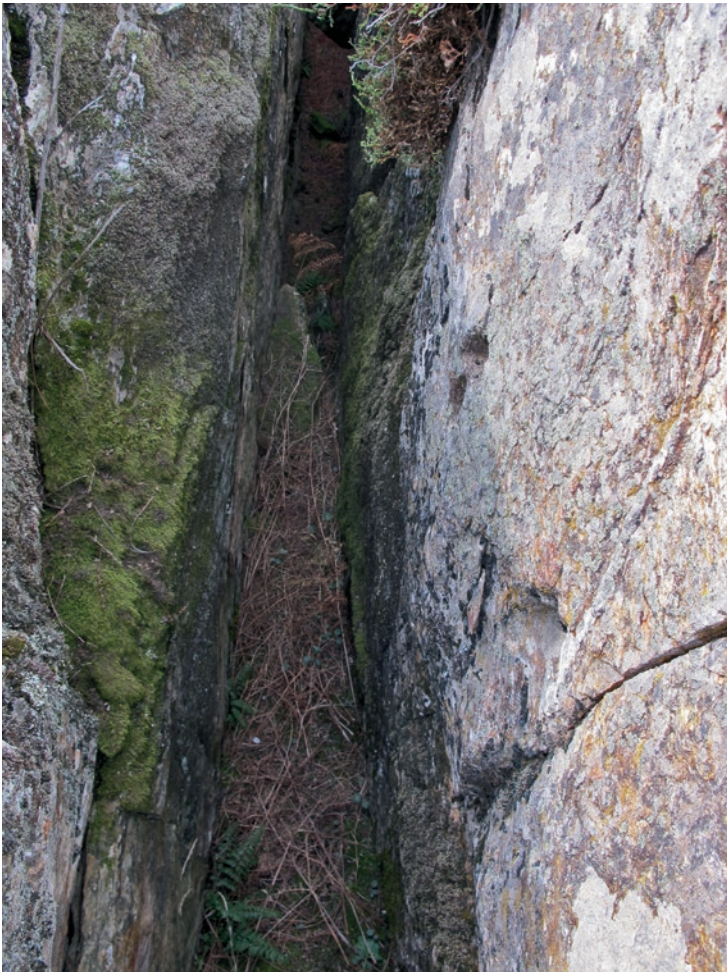
Fig. 3.0-30: Territorium metallorum Tresminas / Jales, Gralheira: extraction zone, not yet completely collapsed with cuts to house the wooden supports (photo: R. Wahl-Clerici).
