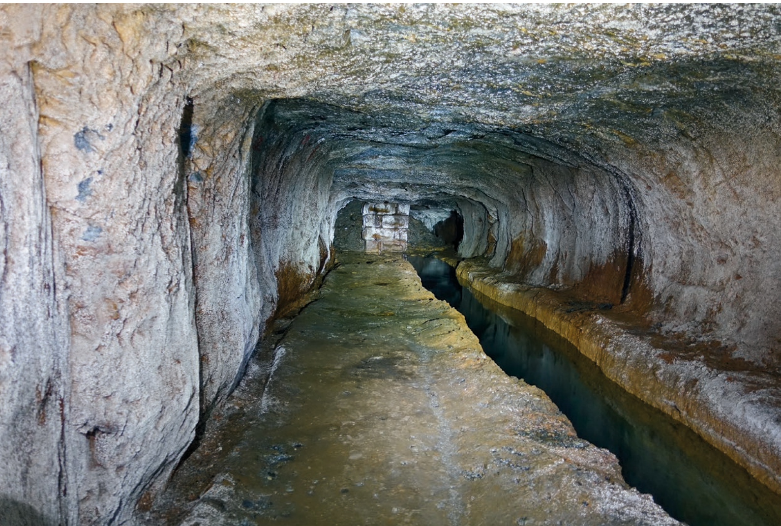
Fig. 3.3-5: Territorium metallorum Tresminas/Jales, Tresminas, Corta de Covas, Galeria do Pilar: view onto the eponymous pillar with the drainage channel along the eastern side (photo: R. Wahl-Clerici).
