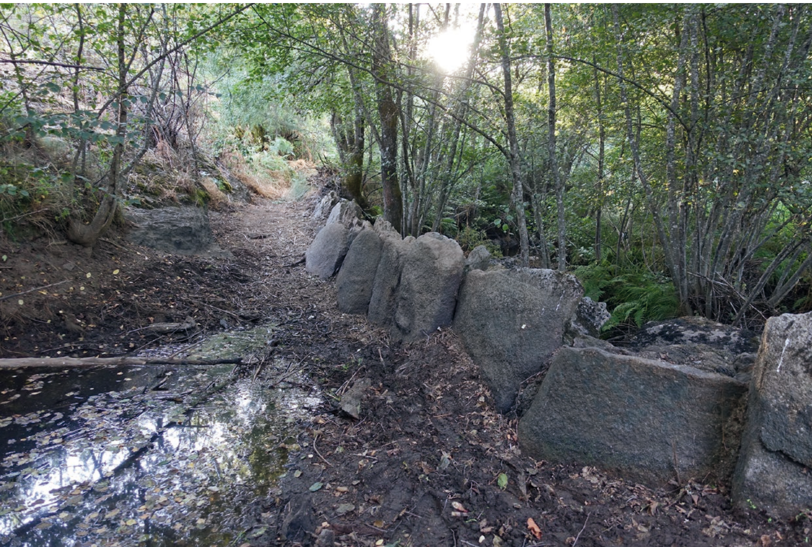
Fig. 5.0-23: Territorium metallorum Tresminas / Jales: weir of the Rio Tinhela in the Vale Curtinhas. View from the north into the reservoir area with the protecting granite slabs, the outlet is marked by the worked rock-part in face of the granite-slabs (photo: R. Wahl-Clerici).
