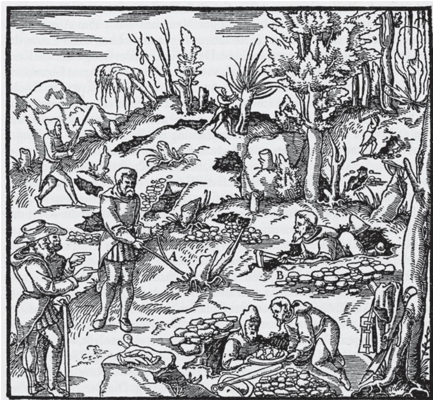
Fig. 2.0-2: Prospection methods after Agricola 1556/1984, 32.
