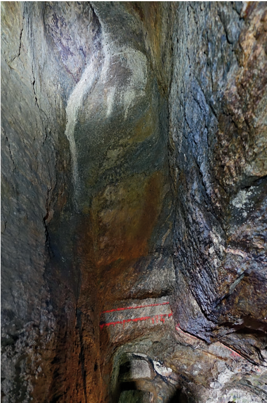
Fig. 4.2-2: Territorium metallorum Tresminas/Jales, Tresminas, Lagoinhos: view into the mining zone inside the mountain of Lagoinhos. It is visible that the abandonment took place in stages. Sample 174 was taken from the deepest step. The southeastern face has broken away at the bottom (photo: R. Wahl-Clerici).
