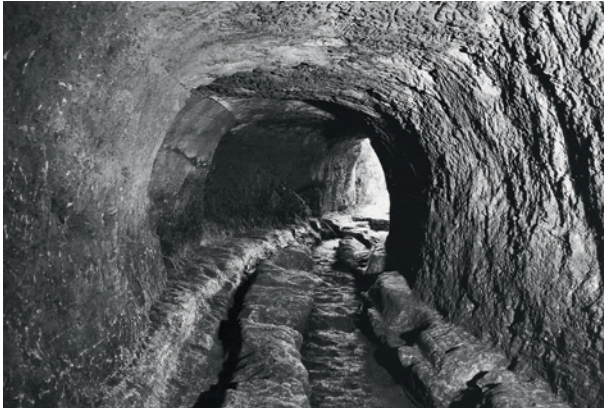
Fig. 3.2-8: Territorium metallorum Tresminas / Jales, Tresminas, Corta de Covas, Galeria Esteves Pinto: the cart tracks and channel and the cuts for the covering of the channel are visible in the floor [FU3/4] (photo: J. Wahl).
