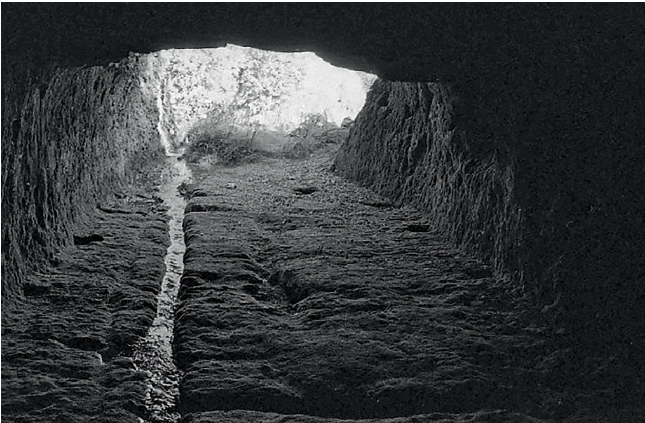
Fig. 3.3-7: Territorium metallorum Tresminas / Jales, Tresminas, Corta da Ribeirinha, Galeria dos Morcegos: tunnel port area with the recesses cut into the rock at the transition from the floor to the sides for the timber props to secure the roof. Also well recognizable is the cut in the floor, in which a votive stone may have been embedded after the abandonment (photo: J. Wahl).
