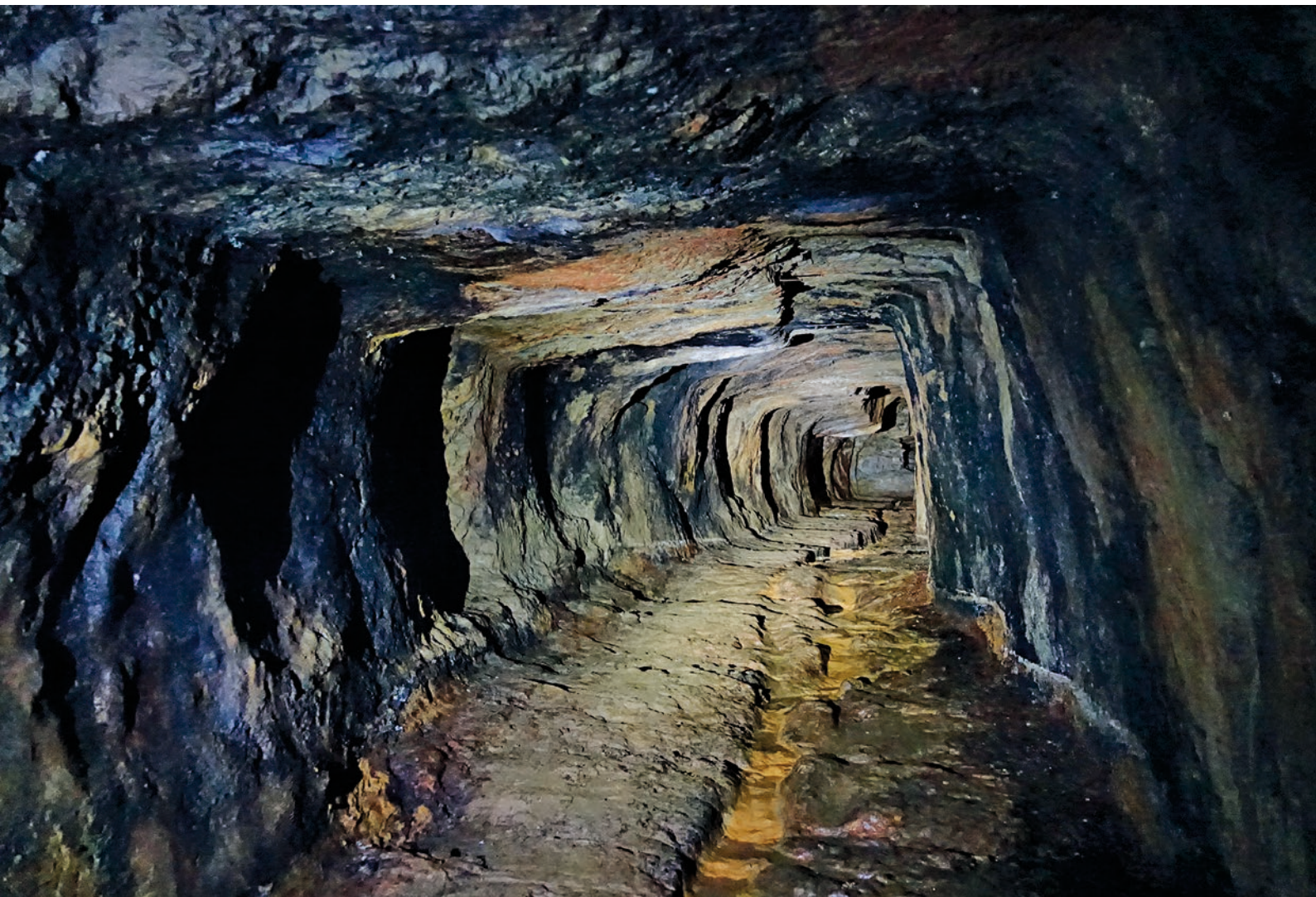
Fig. 3.3.1-19: Territorium metallorum Tresminas / Jales, Tresminas, Galeria dos Morcegos, from the north: in the eastern working faces, both the heading face for widening the cavity and the rock left standing can be seen (photo: R. Wahl-Clerici).
