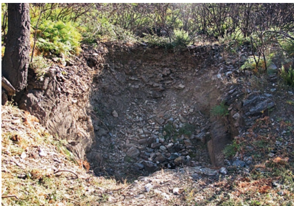
Fig. 3.2-10b: Territorium metallorum Tresminas / Jales, Tresminas, Corta de Covas: view from the north into the former entrance area of the Galeria Jürgen Wahl, completely covered with waste rock material [FU5] (photo: R. Wahl-Clerici).
