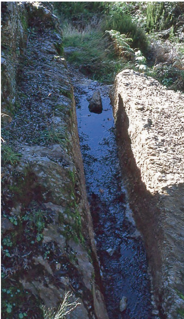
Fig. 5.0-16: Territorium metallorum Tresminas / Jales: detail of the outlet-construction of the dam at the Ribeiro do Muro, southeast of Vilarelho (photo: R. Wahl-Clerici).
