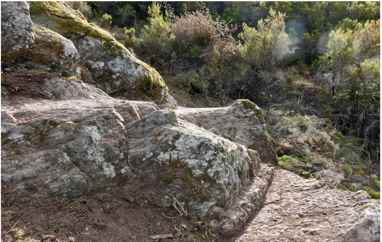
Fig. 5.0-34: Territorium metallorum Tresminas / Jales, Vilarelho: junction of two construction lots on the aqueduct T1 (photo: R. Wahl-Clerici).
