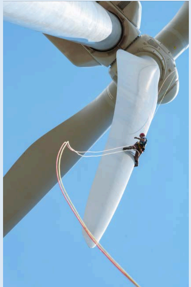
Blade inspection, Colorado
