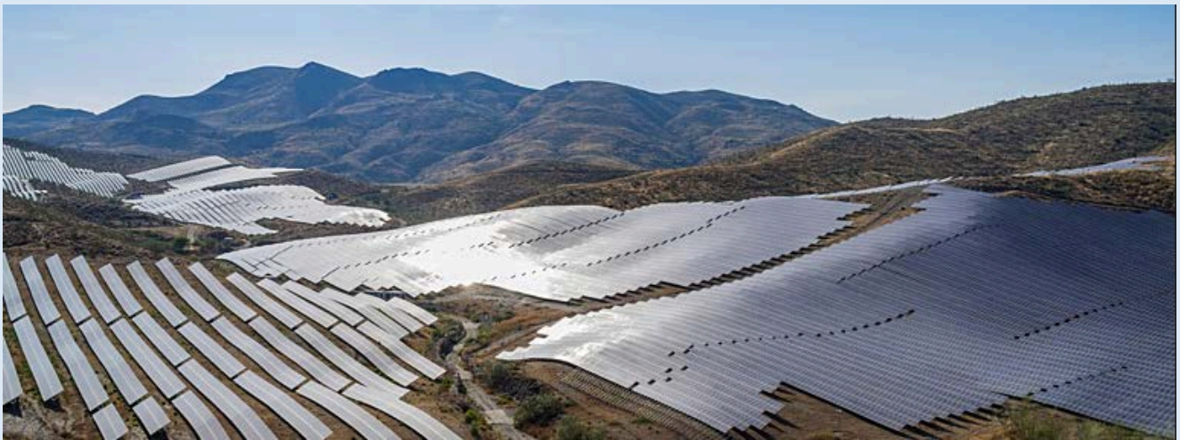
Photovoltaic power station
