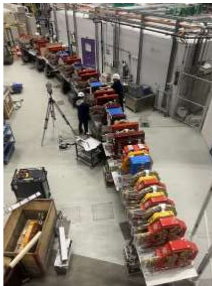
Figure 28: Installation of magnets for upgrading Swiss Light Source SLS to SLS 2.0 [from the presentation of R. Ischebeck].
