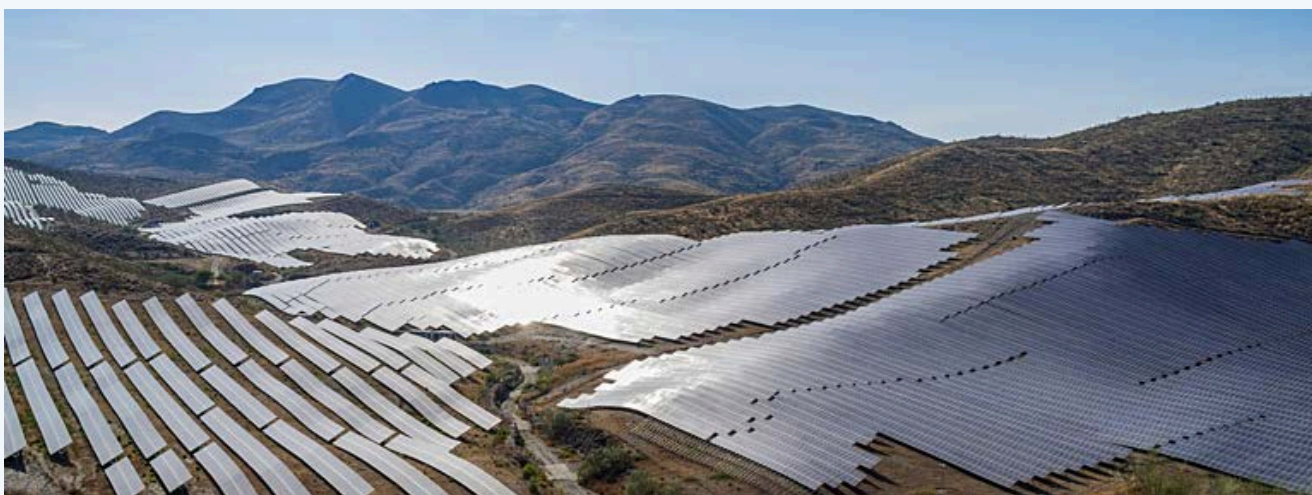
Photovoltaic power station
