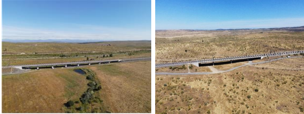
Figure 13 Valdelinares Viaduct, 8 simply supported spans, and La Plata Viaduct, 4-spanned continuous concrete beam
