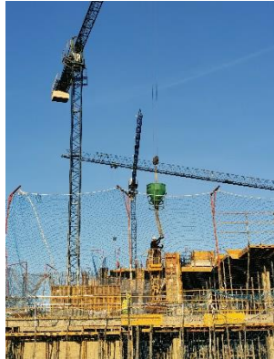
Figure 3 Crane on construction site
