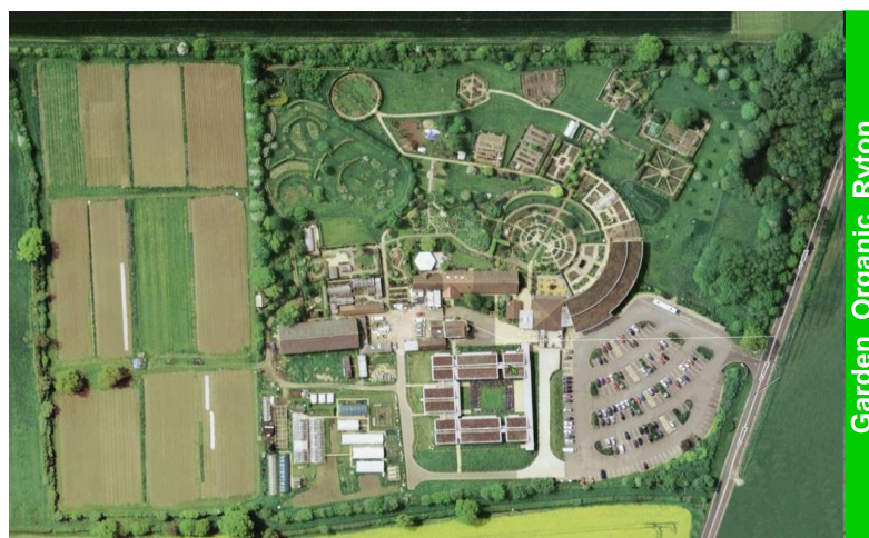
Agenda Item 6: Appendix A Ryton Site Aerial View
