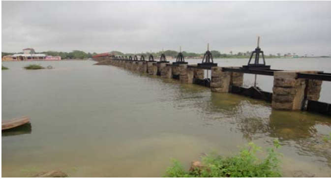
Fig. 2 Existing structures of the Thondamanaru lagoon
