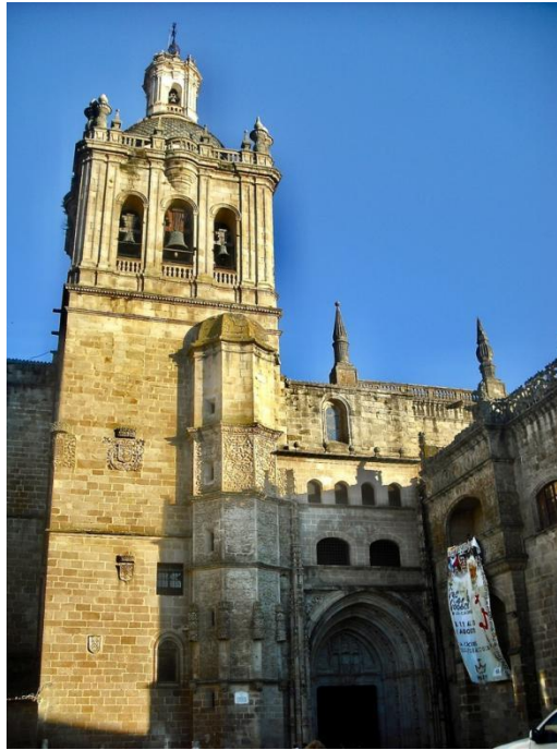
Figure 11. North Façade of the Catedral of Coria in Extremadura. Its construction began between 1495-98, although this gable may have goth or visigothic origins. The case of this cathedral stands as a remarkable example of how one space could be reused throughout different cultural contexts over time. Image: the authors
