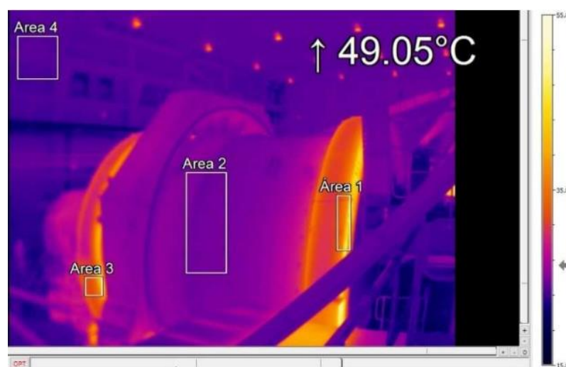
Figure 31: Thermal camera image processing
