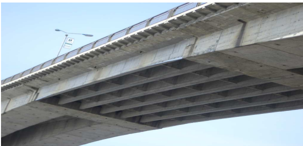
Fig. 1 (c) Hanging beams
