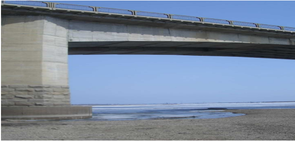
Fig. 1 (b) T-shape cantilever structure
