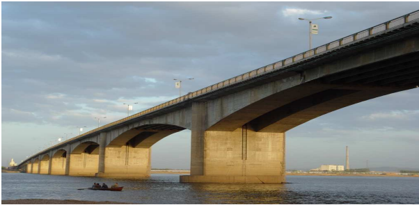
Fig. 1 (a) View of spans
