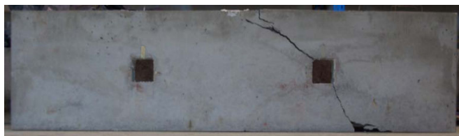
Fig. 11 Crack pattern for beam S05-80-3 [12]
