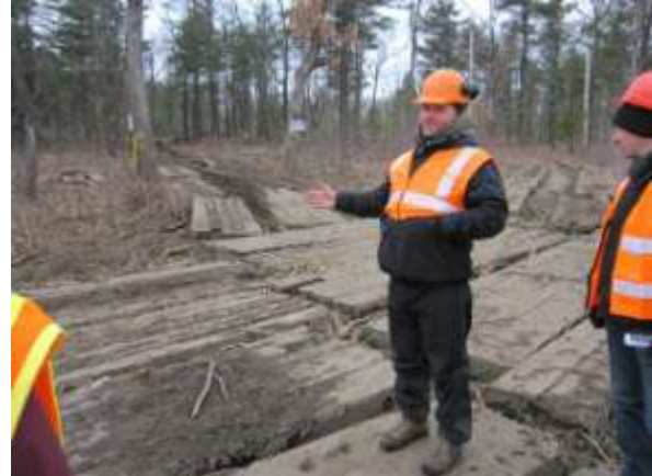
Track laid down to allow forestry work
