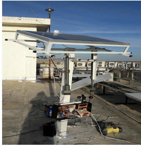
Figure 23: Project on university roof
