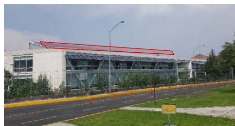
Fig. 3 Photography of the C3-UNAM Building rooftop PV System, University City. Image by Viridiana Ardura Perea
