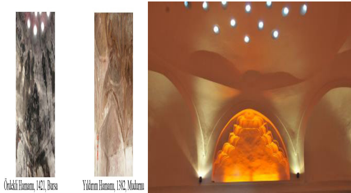
Figure 10. Examples of diamond shaped (baklava) tromp (Yıldırım Bathhouse, Mudurnu) and tromp with muqarnas (Ördekli Bathhouse, Bursa)
