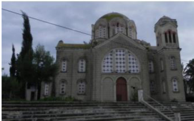
Figure 2. An example of a dome sitting on a circular pedestal (Yüceer, 2016, p. 444)
