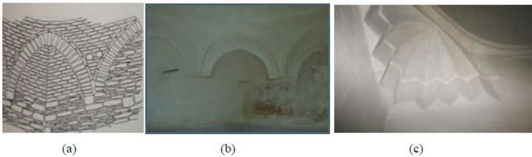
Figure 8. Drawing and application examples of simple, edged and grooved tromps (a) Drawing of an edged tromp (b) An example of simple tromp: Mevlana Bathhouse, Tokat (c) An example of grooved tromp: Mustafâ Bey Bathhouse, Amasya (Aktuğ, 1989).
