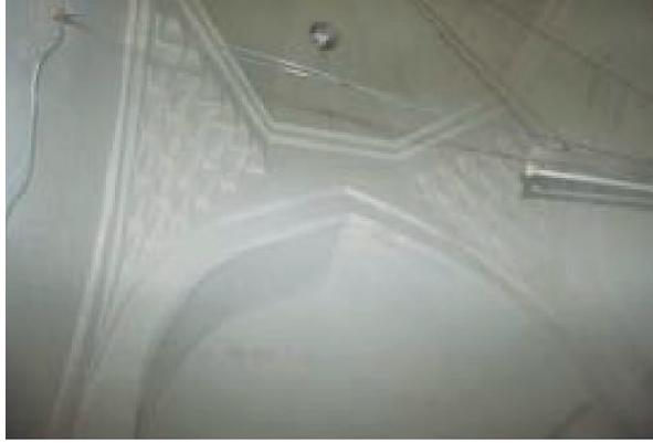
Figure 25. An example of plane triangle with muqarnas type: Orta Bathhouse, Bolu, 1389
