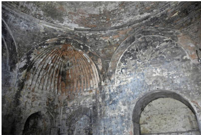
Figure 11. An example of grooved tromp: Sokullu Bathhouse, (Aktuğ, 1989).
