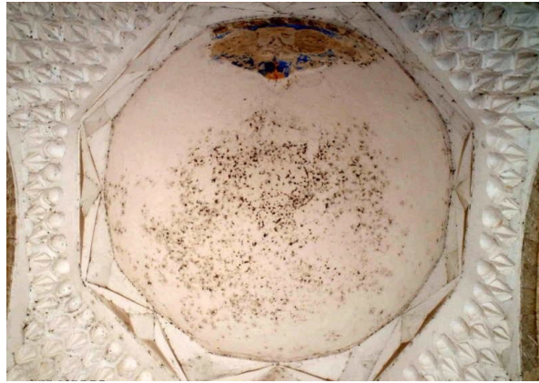
Figure 17. An example of muqarnas as a transition element between dome and bearer dome.
