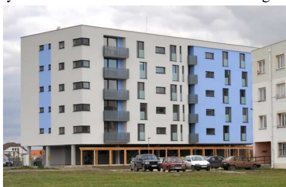
Newly erected residential building connected to the extended geothermal district heating loop at Galanta
