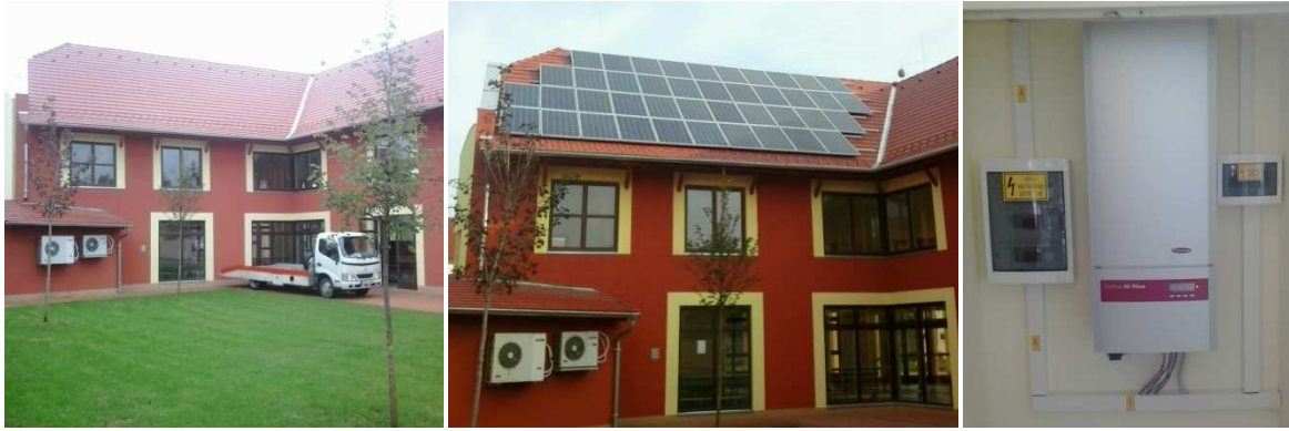
Solar PV panels before and after installation to supply the LED public lighting system
