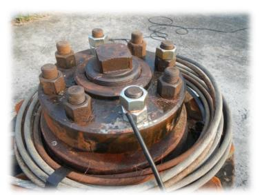
Figure 14 : Borehole head with electrical connection.
