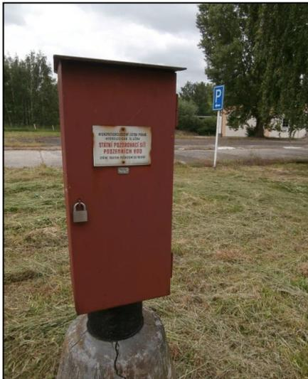
Figure 18 - TH-10 borehole, 500 m deep, Predlice.
