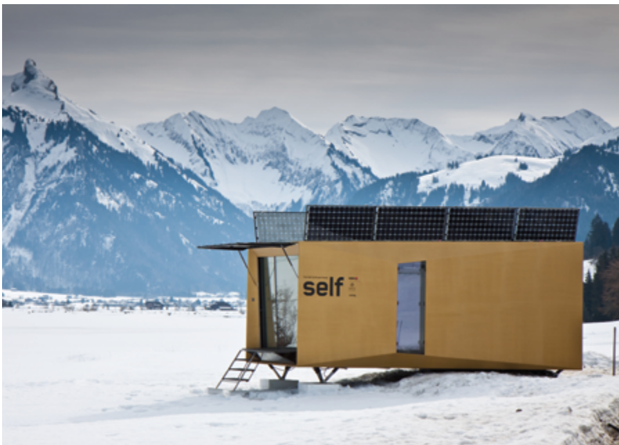
← Testing the Self, an earlier Empa and Eawag collaboration, 2010. The self uses gravity driven membrane for its water treatment. Photo Beat Geyer, Empa.
