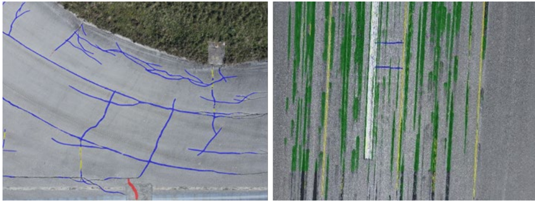
Figure 3 Results of the deployed DDCV method. Cracks are highlighted with red, joints with blue, construction joints with yellow and tire marks with green colour, respectively (Krestenitis&Ioannidis, 2022).
