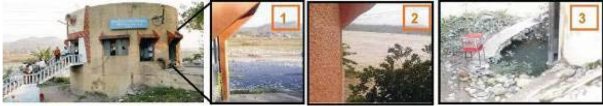
Figure 6-10 RBF well IW 24 in Haridwar (left photo), (1) view of the Ganga River in the background in April 2005 (pre-monsoon), (2) flood-water of Ganga inundates the base of well on 19/09/2010 and (3) damage by scouring to base of well no. 24 (photos from L to R: Schoenheinz and Grischek (2005), Subodh & Kumar (2010))
