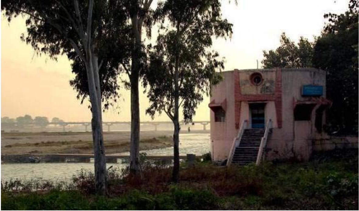
Figure 6-7 Example of large-diameter RBF well adjacent to Ganga River, Haridwar (Photo: L. Rossoff, HTWD, 2011)
