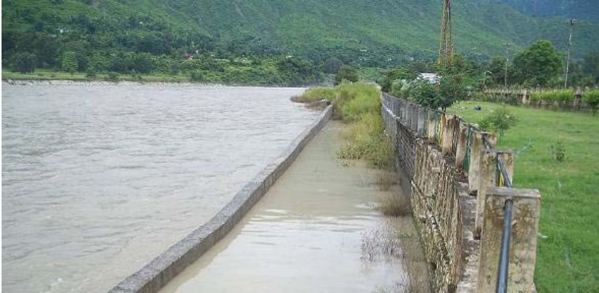
Figure 3-10 View of flood-wall (left) and retaining wall (right) of the lower level of the park where the RBF site in Srinagar is located (Photo: M. Ronghang, IITR, 2011)
