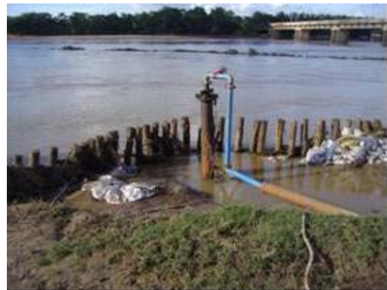
Figure 3-14 A RBF well in Kharagpur (Kangsabati River, West Bengal) at risk of contamination by floods (Photo: C. Sandhu)
