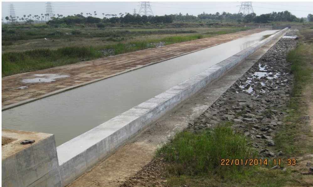
Figure 11 Photograph of Check dam at Irulipattu-view from up stream
